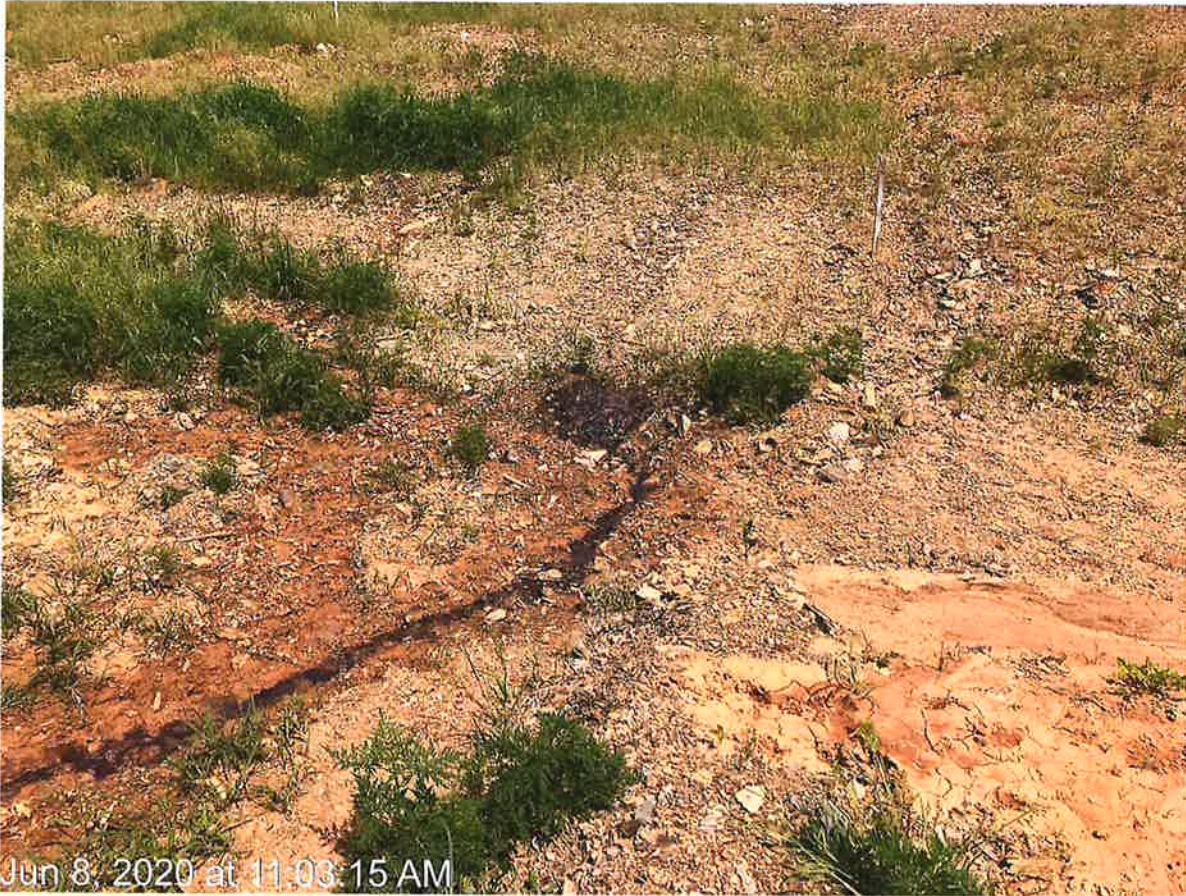
Figure 6 - Leachate outbreak and stream on southeast facing slope
