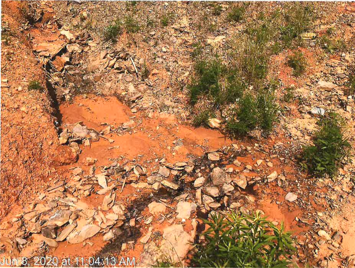
Figure 2 - Leachate outbreak on southeast facing slope
