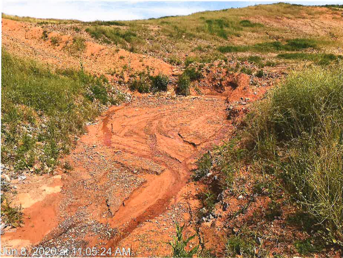
Figure 1 - Leachate stream on southeast facing slope
