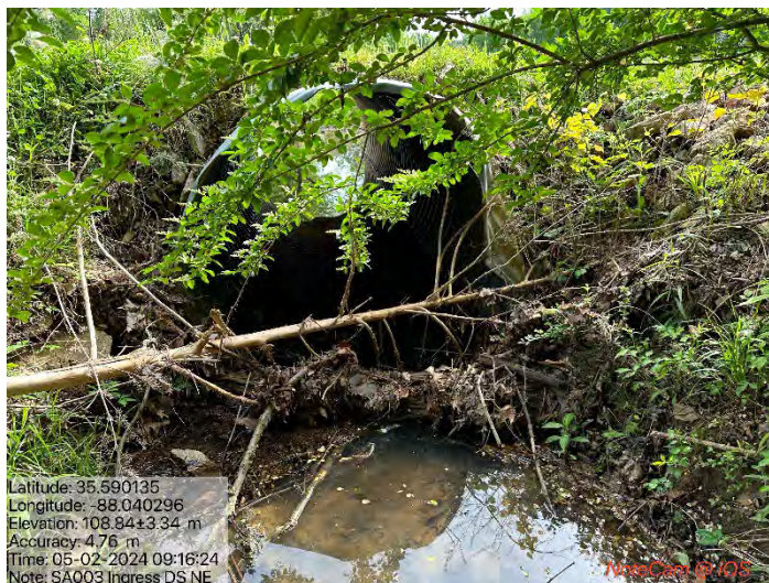
Figure 17. Intermittent stream SA003 ingress; view facing northeast downstream.
