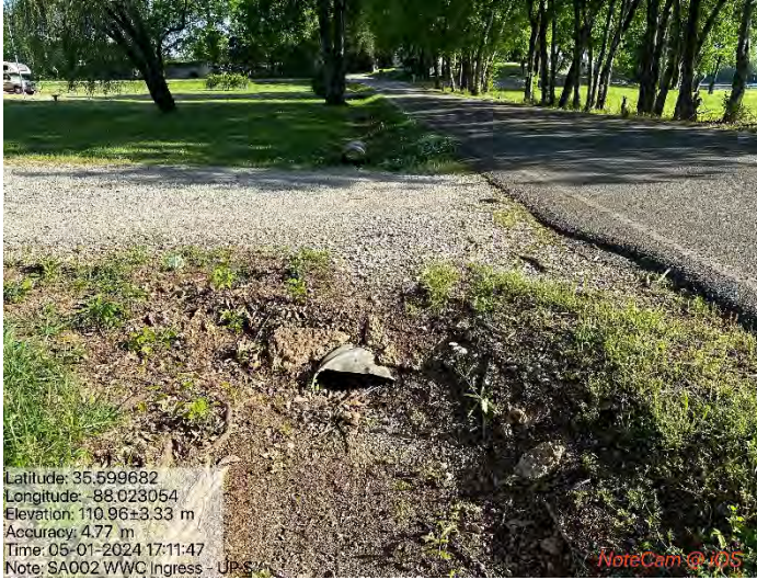
Figure 18. Wet weather conveyance SA002 ingress; view facing south upstream.
