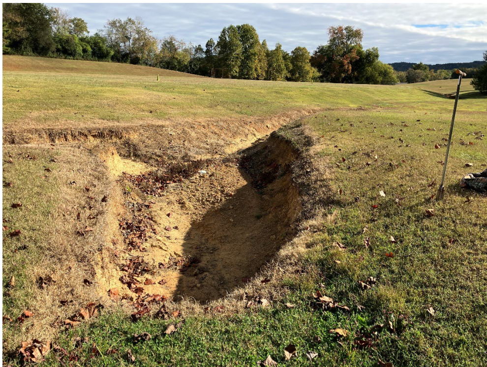
Photo 2: View at start of WWC-1/UDF-1 facing downstream located at 35.8824776, -84.6210053.
