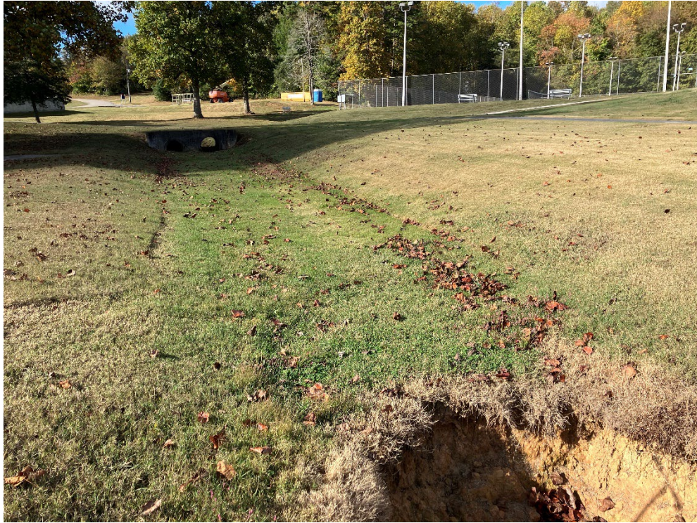
Photo 1: View at start of WWC-1/UDF-1 facing upstream located at 35.8824776, -84.6210053.
