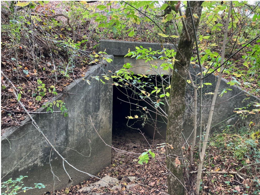
Photo 6: View at end of WWC-2/EPH-1 facing downstream located at 35.8839929, -84.6176475.
