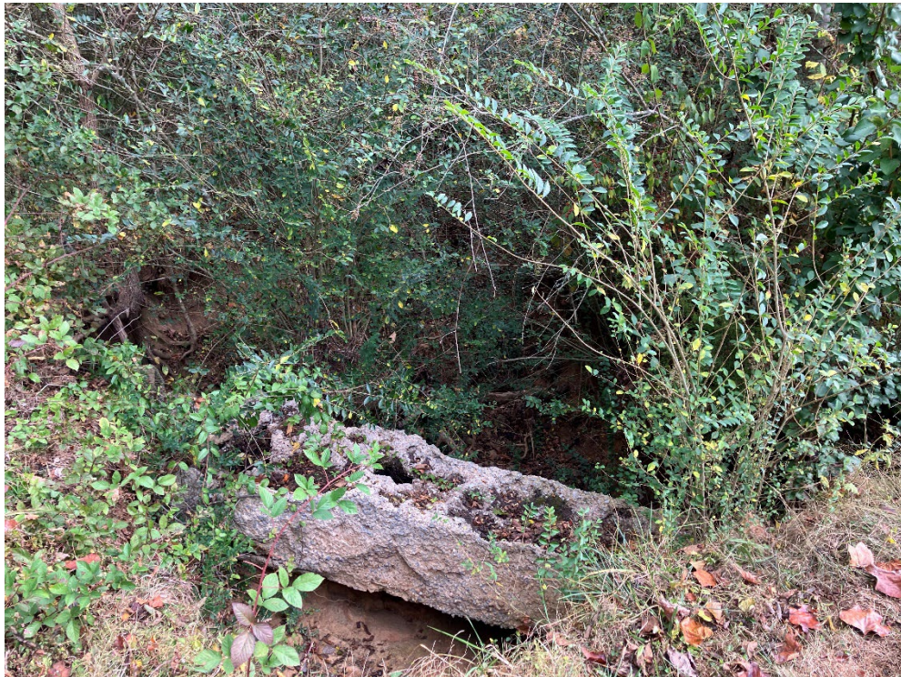
Photo 4: View at end of WWC-1/UDF-1, start of WWC-2/EPH-1 facing downstream located at 35.8837337, -846178658.
