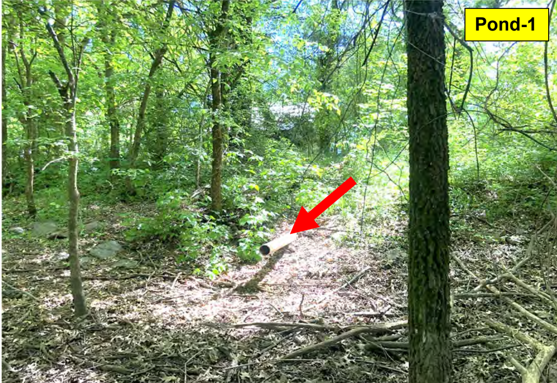
Photo 5 – View of 4-inch pipe leading into the pond from the adjoining property to the east.
