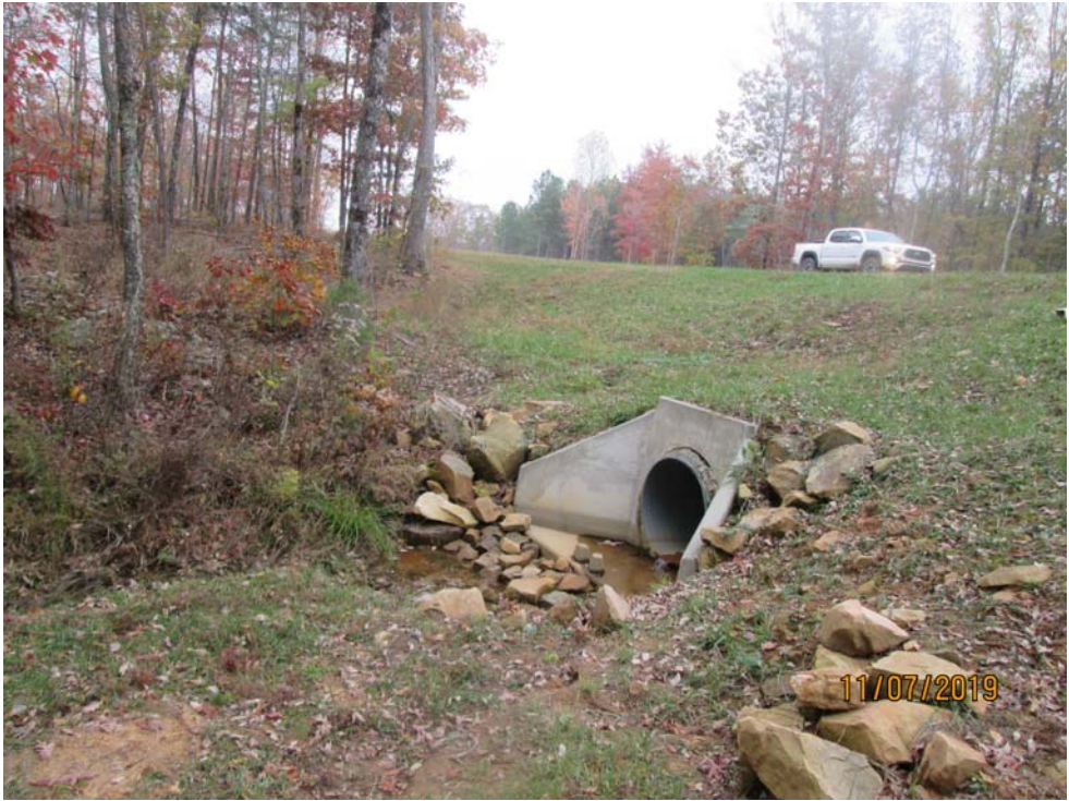
Photo 3: Minor Road Crossing #2 View of the stabilized downstream end of the road crossing. Photo Taken 11/7/2019
