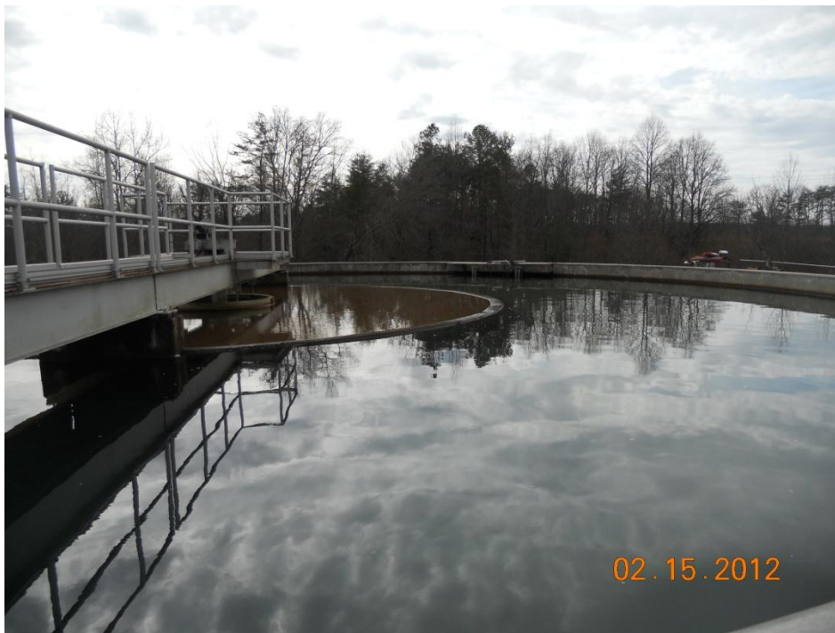
Settling basin prior to beginning discharge
