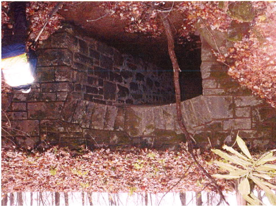
View of Channel, Upstream of Culvert
