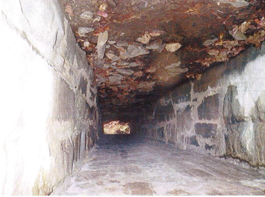
View of Culvert Channel, Looking Upstream
