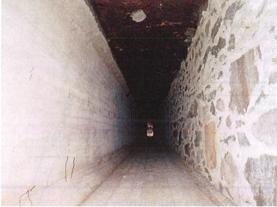
View of Culvert Channel, Looking Downstream
