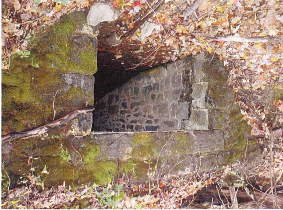
View of Channel, Downstream of Culvert
