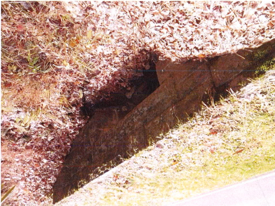
View of Culvert, Upstream
