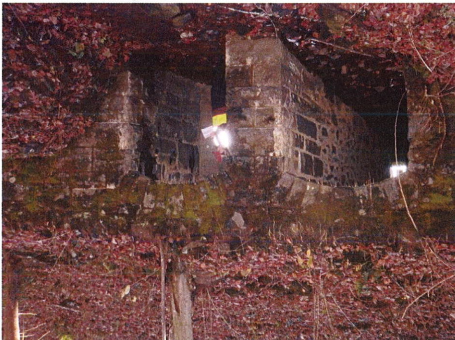
View of Channel, Downstream of Culvert
