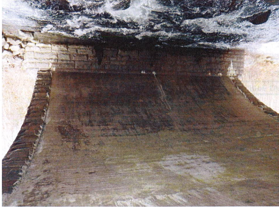
View of Main Channel Crossing (South Span)
