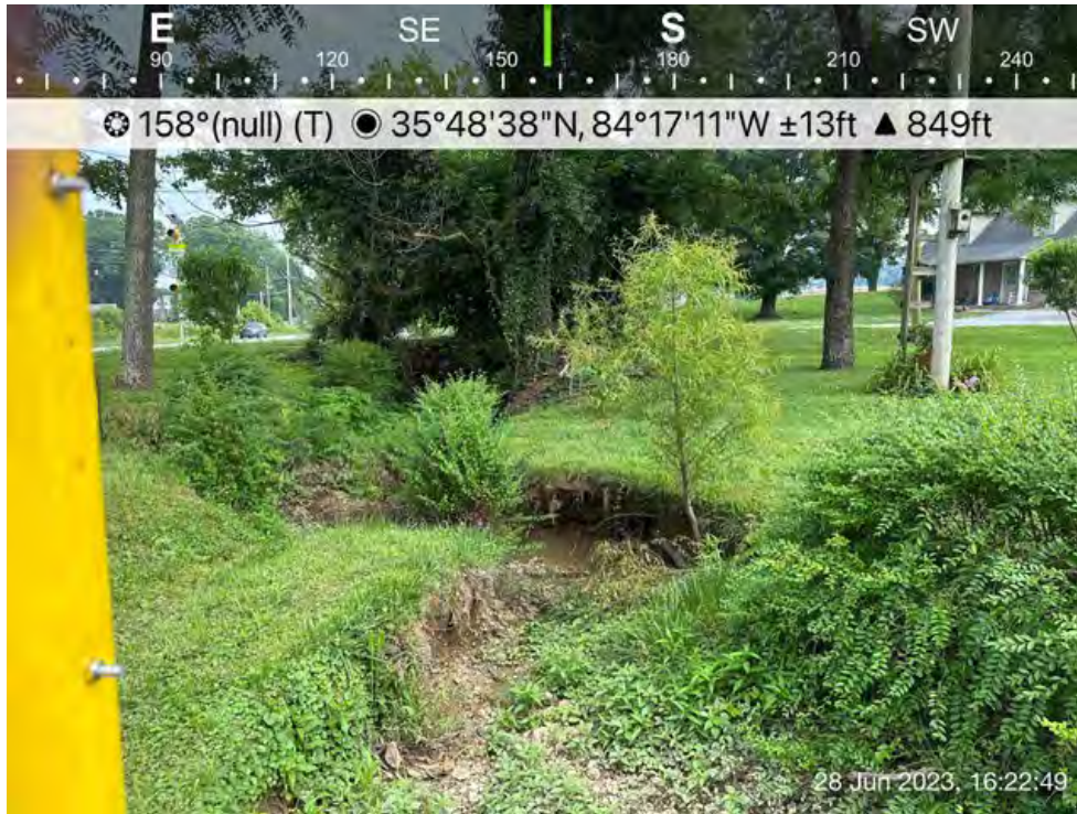
Photo 5- Facing downstream from pipeline.
