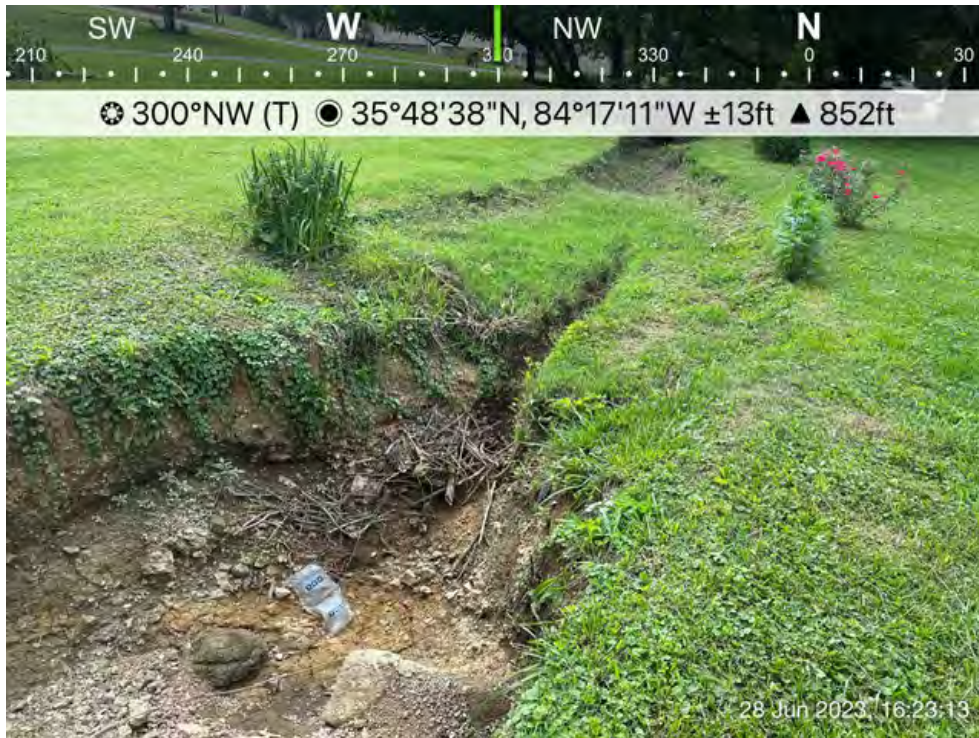
Photo 3 – Facing upstream at the exposed pipe location.
