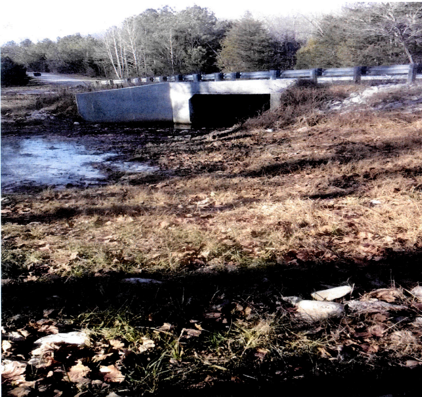
Upstream end of new box culvert
