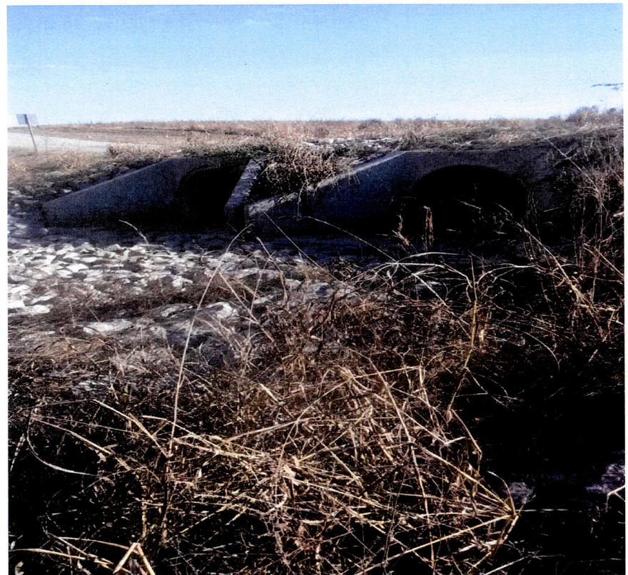
Downstream end of new culverts
