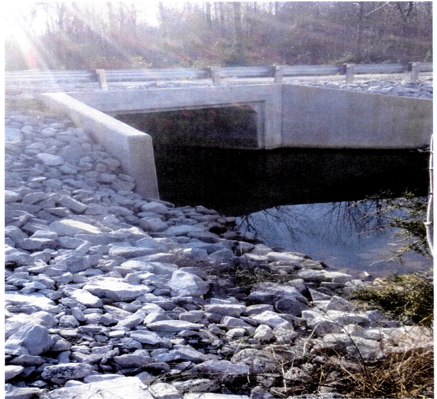
Downstream end of new box culvert
