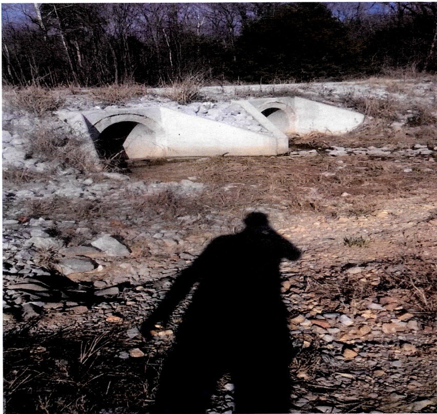
Upstream end of new culverts
