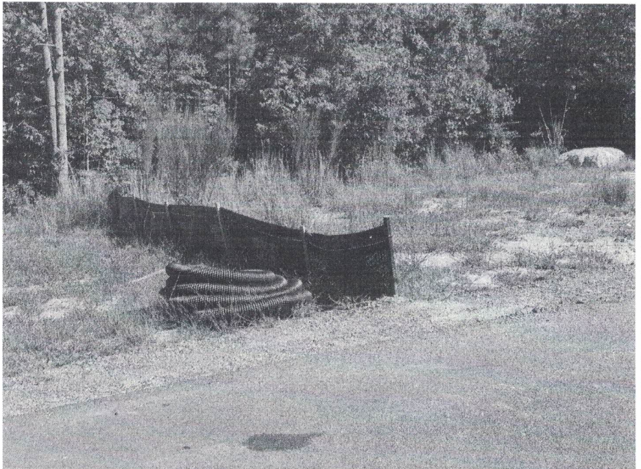
Photo 6: Outfall S208 An individual home construction site was observed, and erosion control measures appeared to be in place and functioning properly. Photo Taken 8/31/2023
