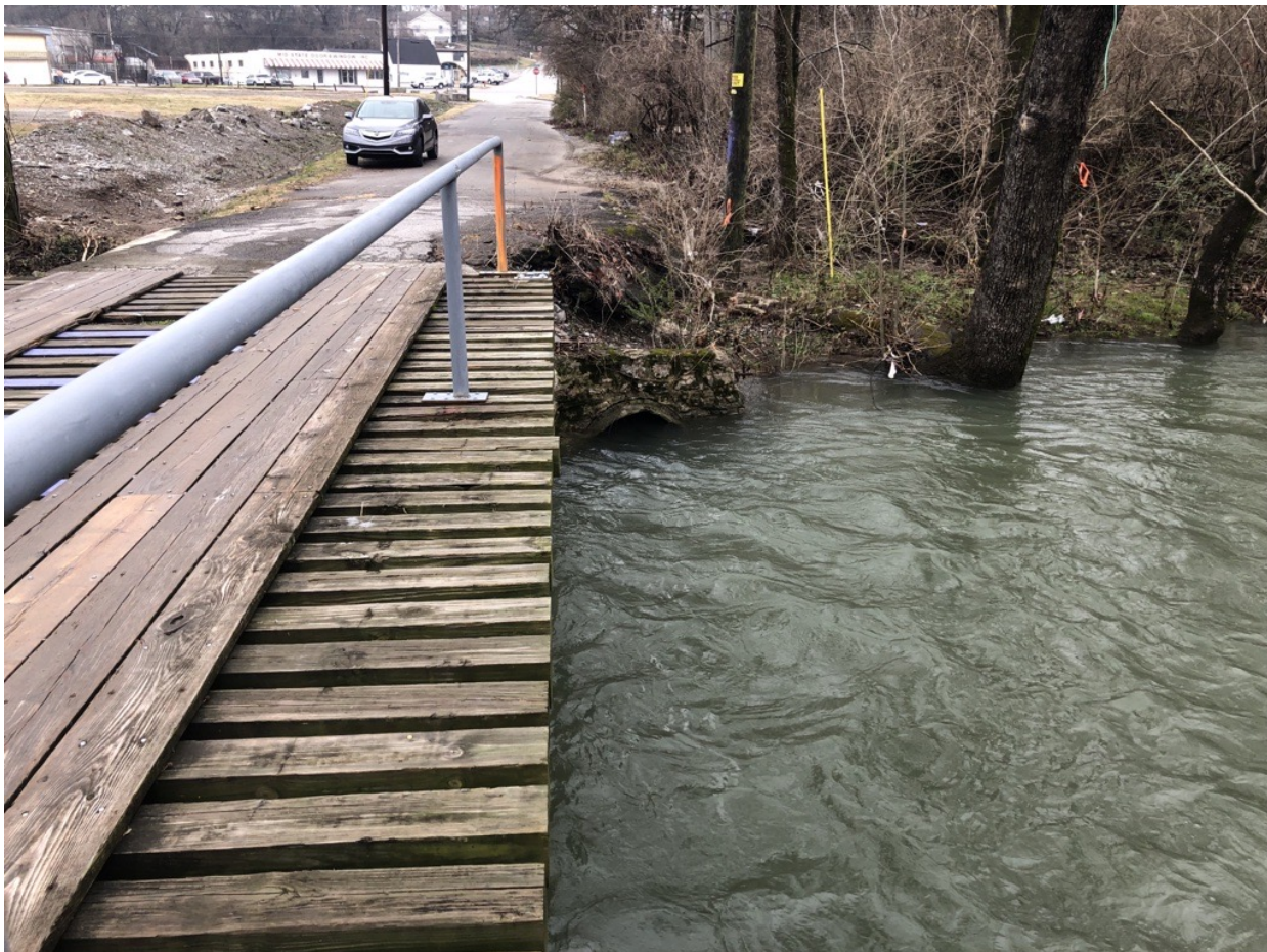
EXISTING STORMWATER OUTFALL - LOOKING WEST FROM MOORE AVE. BRIDGE
