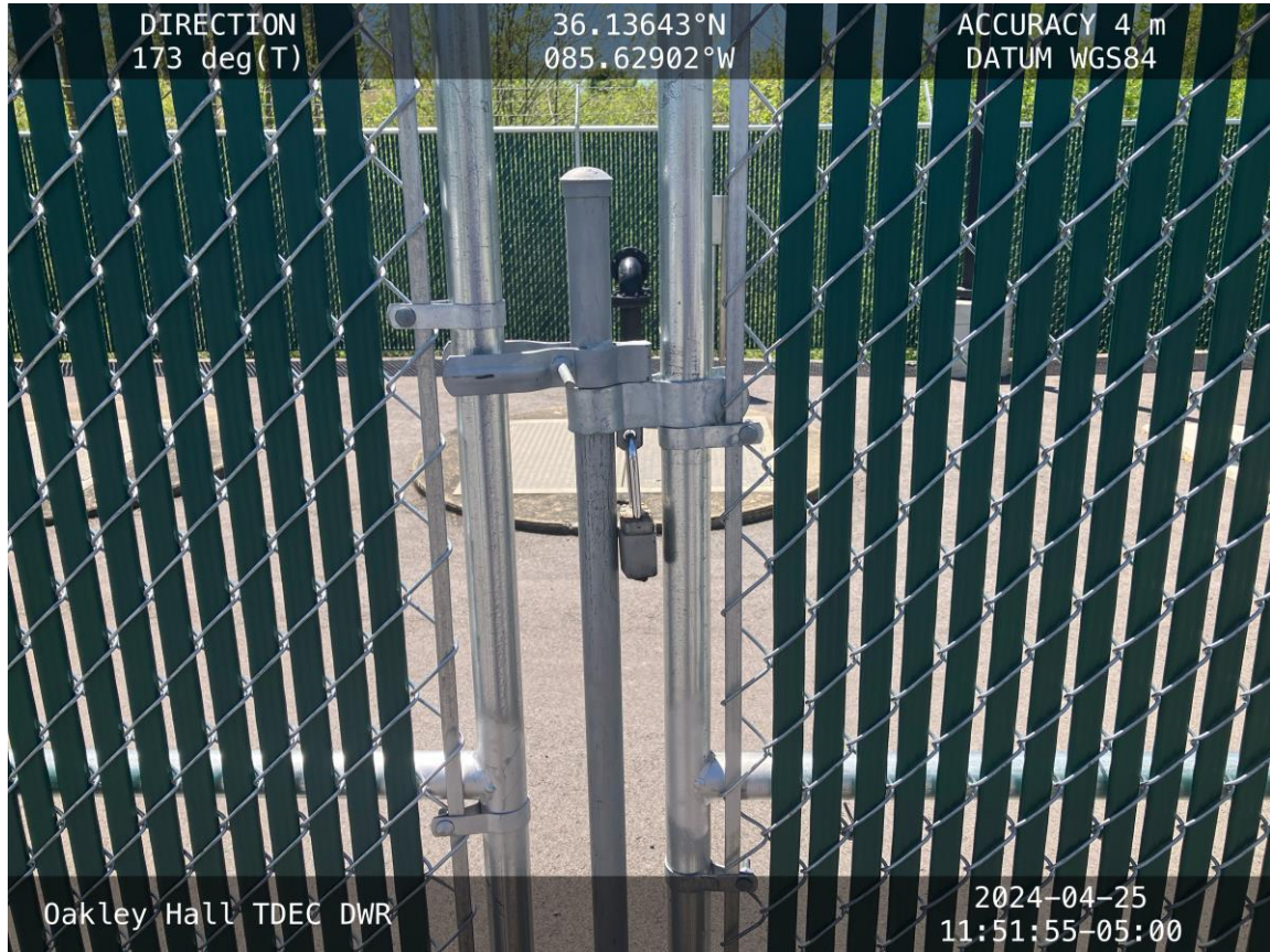
Security at the two pump stations was discussed. A chain should be added at this gate to reduce the possibility of unauthorized entry. Photo By: Oakley Hall, April 25, 2024
