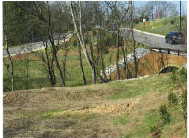
Site updates and drainage stable
