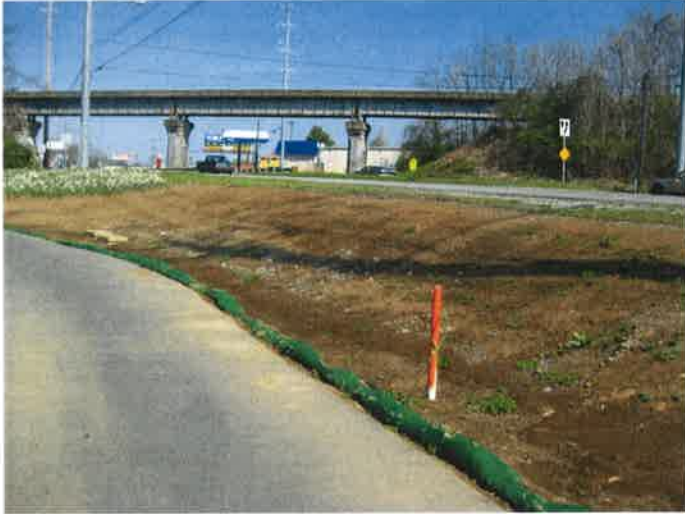
Filter sock in place until grass grows
