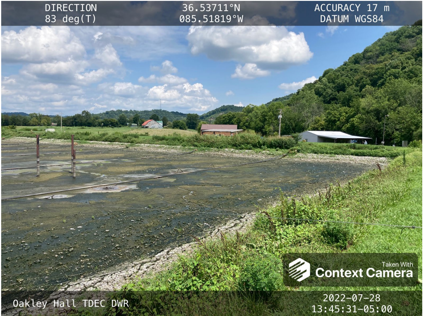
The sludge buildup in the ponds has likely affected the efficiency of the aeration unit(s).
