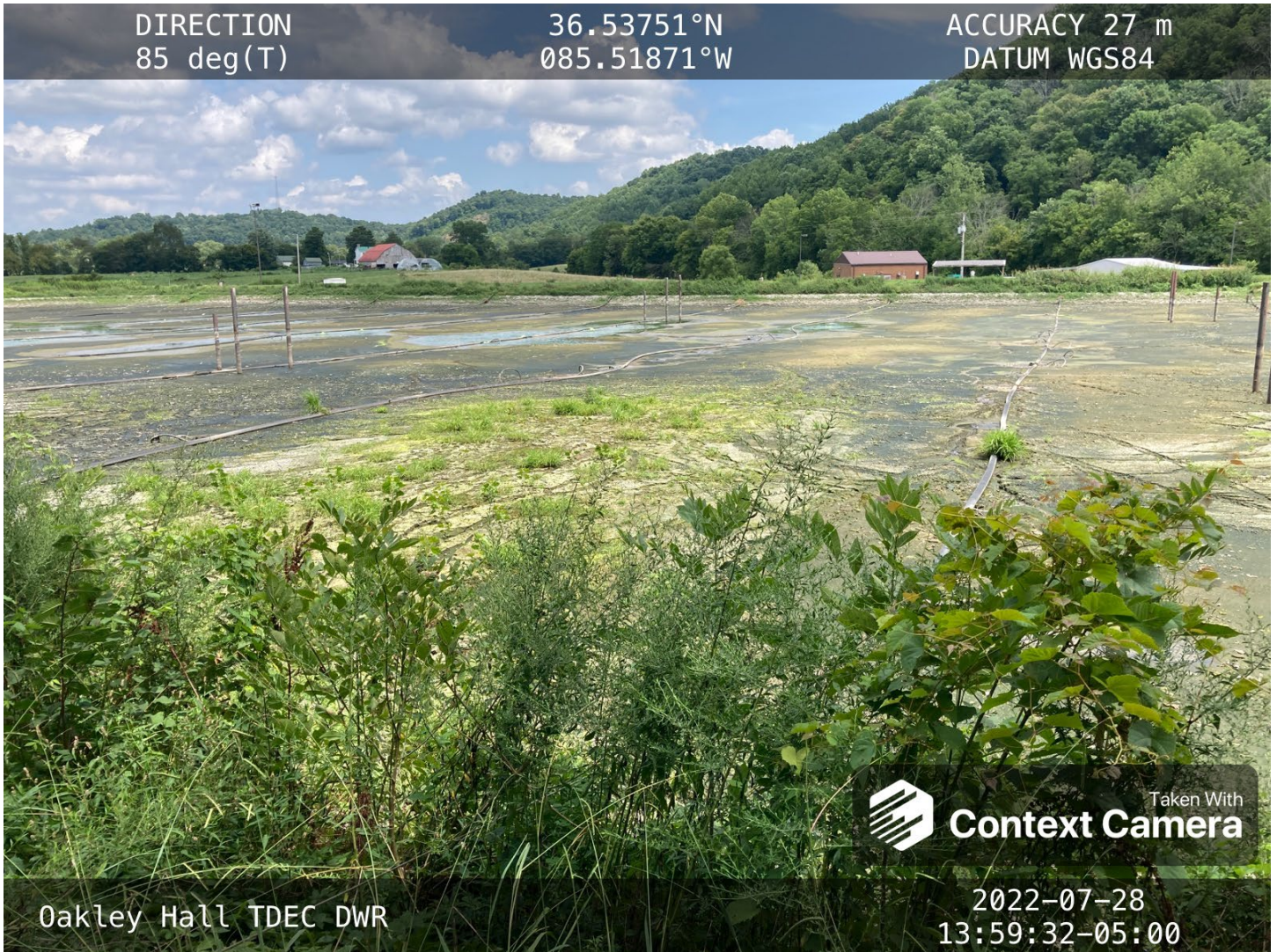
The first pond is pictured. Note the solids delta with vegetation in the forefront of the picture. This material should have never been allowed to build up in the pond. This is due to a lack of proper maintenance by periodically removing the solids.
