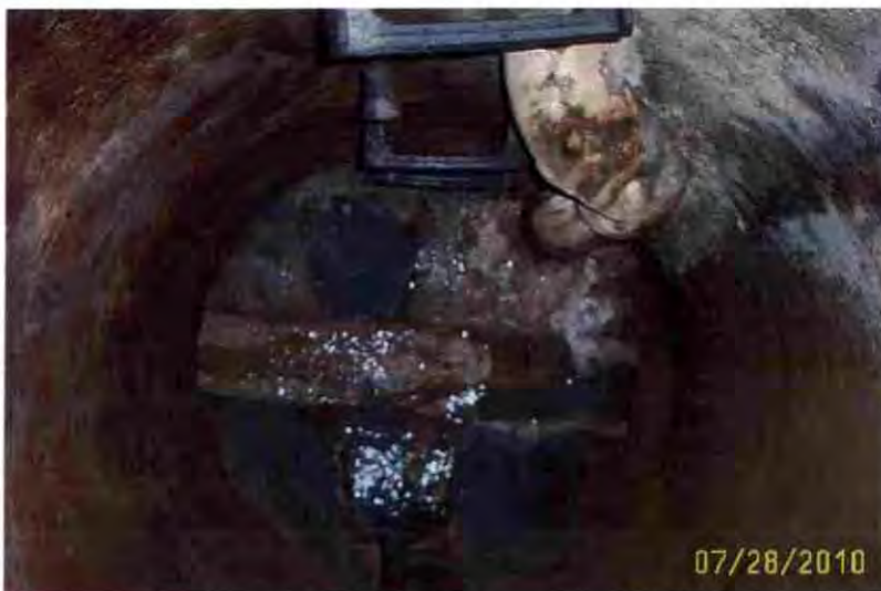
Outback discharge to the City Sewer (7/28/10)
