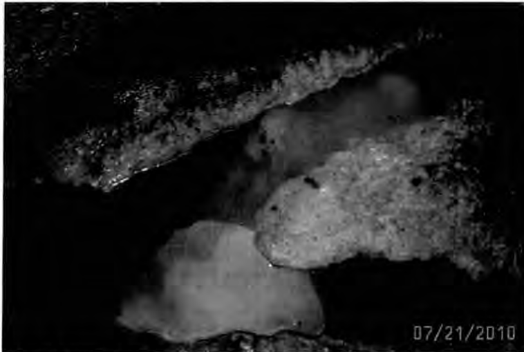
First downstream manhole from Vittles
