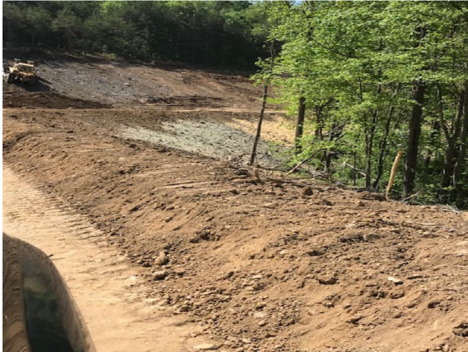
Pic 14 Berm at closing end of job-timber separated and hydro seeded (5-5-22) Ditch to 103
