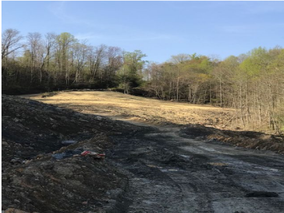
Pic 7 Upslope of Pond 100 (was supplemented with hydro-seeding after this 4/22/22)
