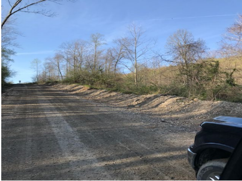
Pic. 2 Haulroad Berm Repair near top
