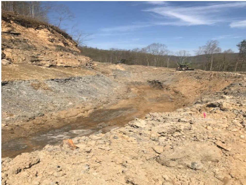
Pic 11 Pond 103 during construction with initial clay liner material being placed (4-22-22)
