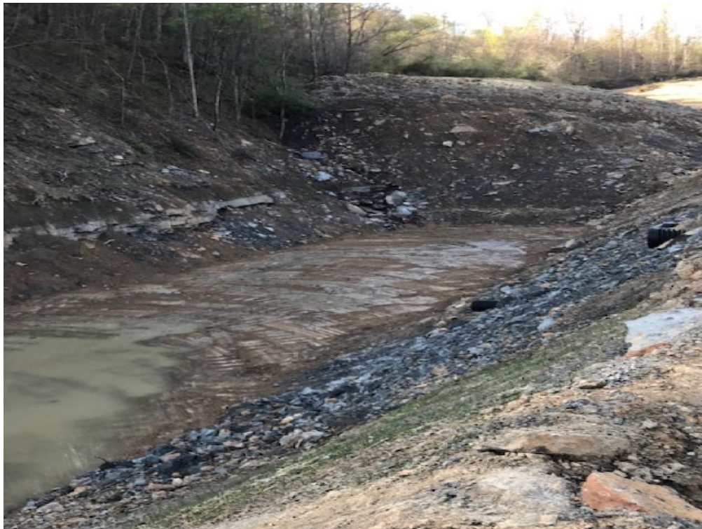
Pic 5 Pond 100 bottom seal and auger hole seal (background)
