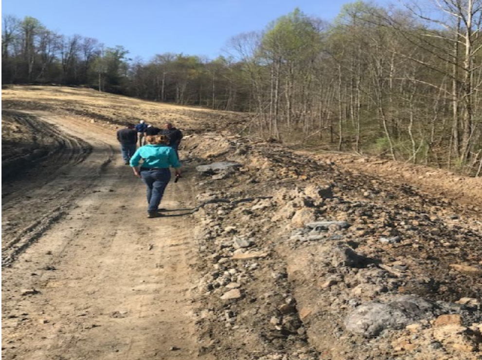
Pic 8 Field walk of Pond 100, upslope ditch, upslope area (4-22-22)
