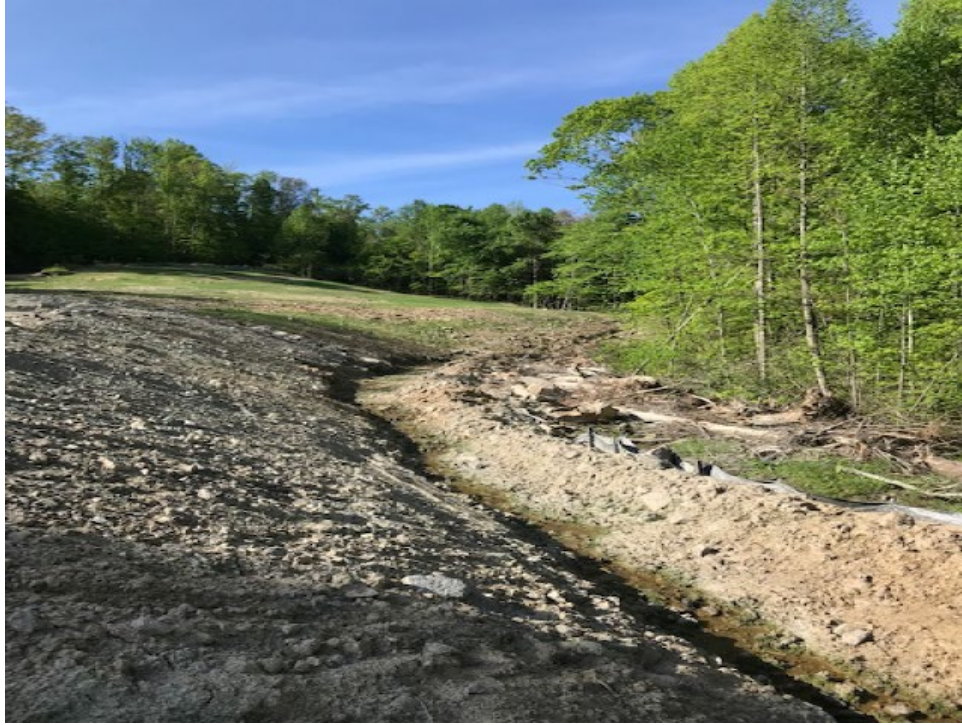
Pic. 12 Vegetative Growth on Hydro seeded areas-ditch repair(5-5-22)
