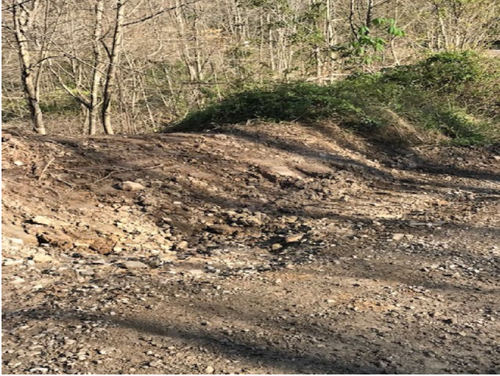
Pic. 1 Haulroad Berm Repair
