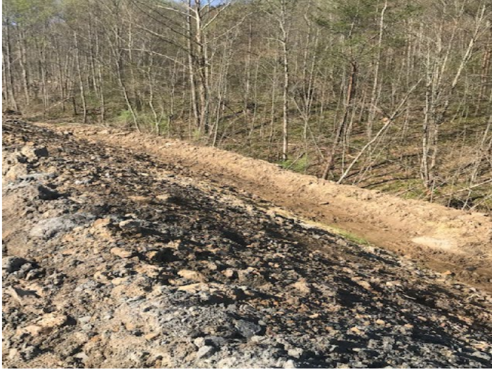
Pic 6 Re-Worked Ditch to pond 100
