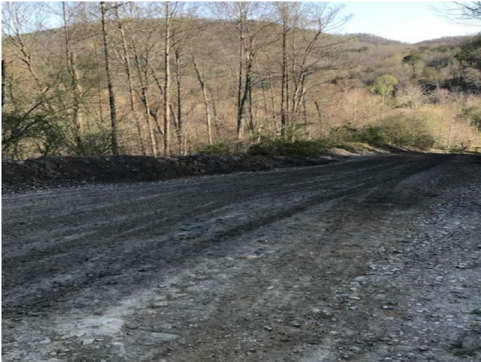
Pic. 3 Haulroad Berm Repair looking down
