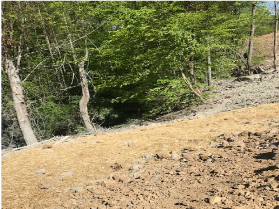
Pic 15 Berm graded, timber separated view toward end of job (5-5-22)
