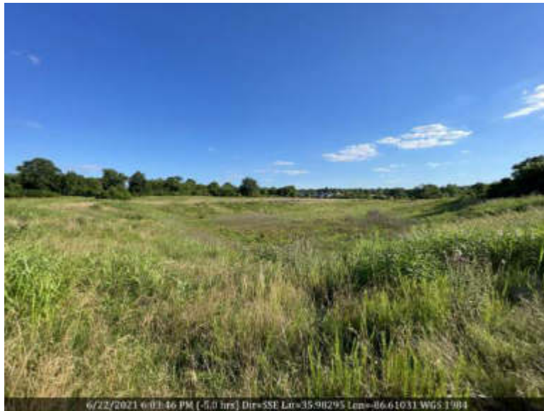
14 Overview of large detention pond, facing southwest.
