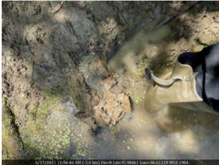
26 View of clay liner in ISOPND-A.
