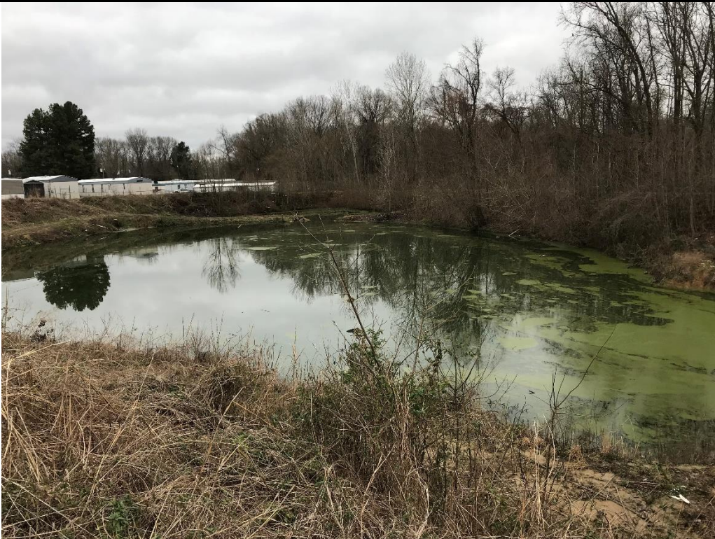
Photo 3. View of the northern portion of the wastewater treatment lagoon. The aerator serving the northern portion of the lagoon was inoperable during the inspection.
