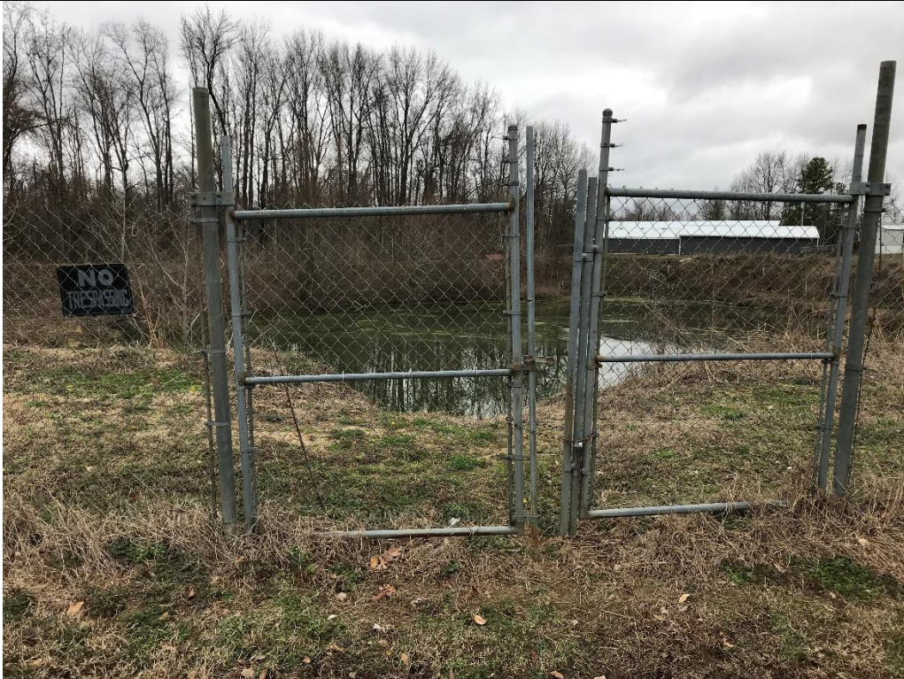
Photo 6. Secured gate and "No Trespassing" sign at the entrance of the wastewater treatment lagoon. The appropriate sign was not posted at the entrance of the wastewater treatment lagoon.
