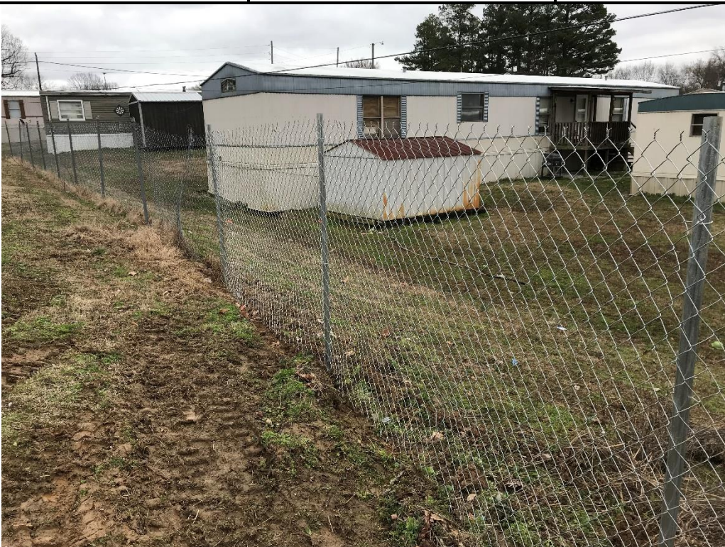
Photo 4. The portion of fencing that was less than 4 ft. high observed during the previous inspection had been replaced with appropriate fencing.
