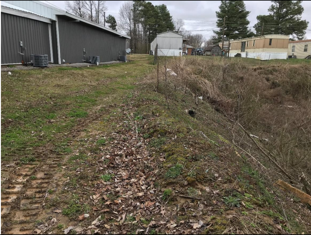
Photo 5. There is a berm that surrounds the top of the lagoon which prevents rainwater from entering.
