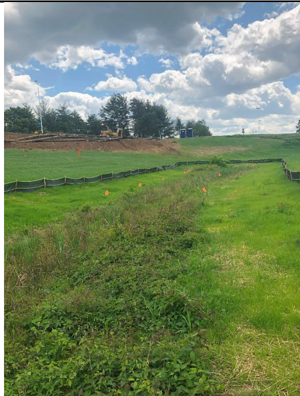
Photograph No. 4: Southeast facing view emergent wetland 3 (W3) CPC's existing ROW.
