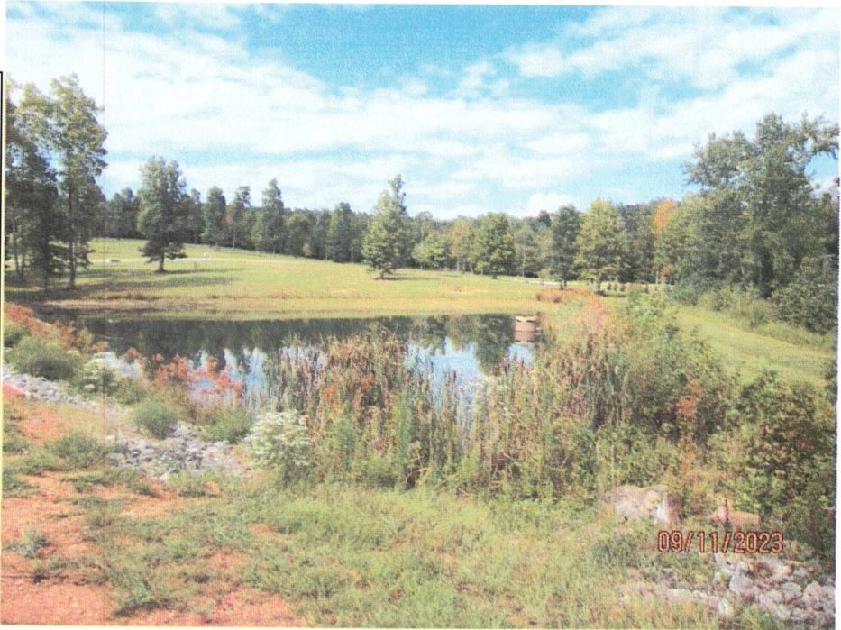
Photo 2: Outfall S66 A stormwater basin has been installed and appears to be functioning properly. Photo Taken 9/11/2023
