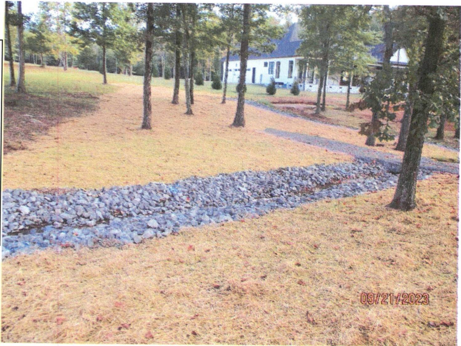
Photo 2: Outfall S66 The individual lot level erosion controls have been installed and appear to be functioning properly. Photo Taken 9/21/2023
