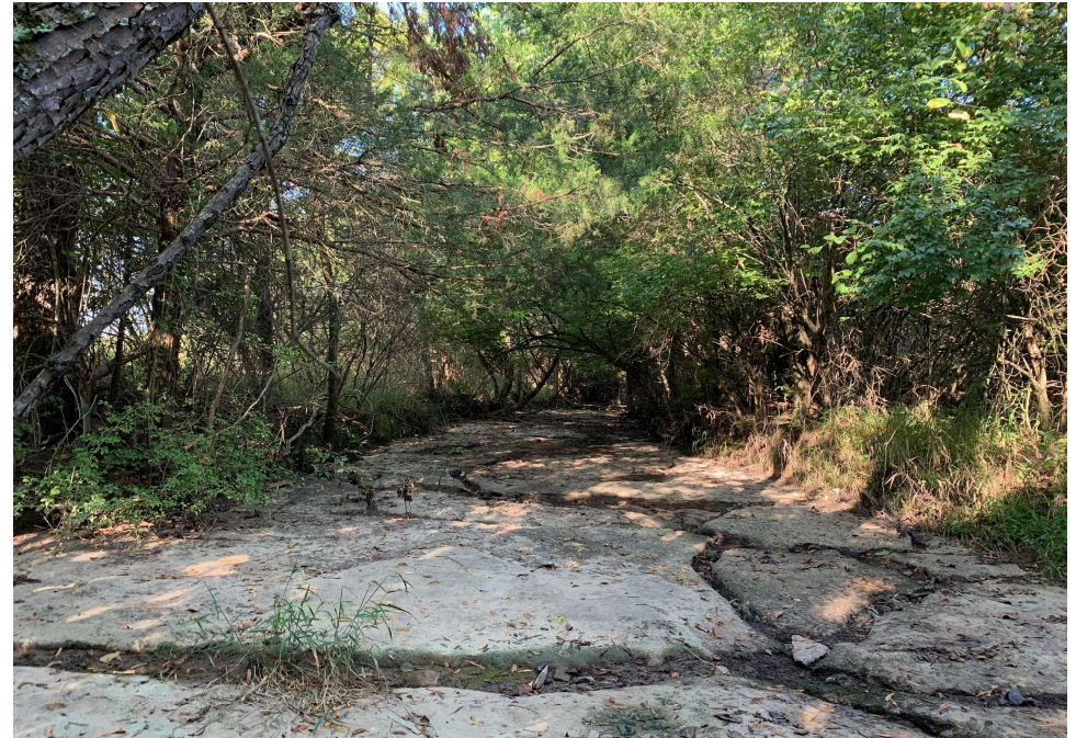
4. Facing Upstream (Westerly) [35.9835°, -86.6085°]
