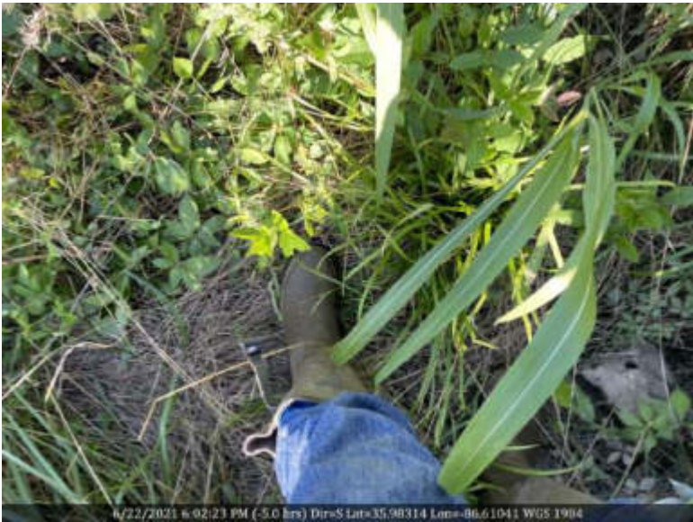
13 View of substrate and vegetation in D-1 below culvert outlet, facing down.
