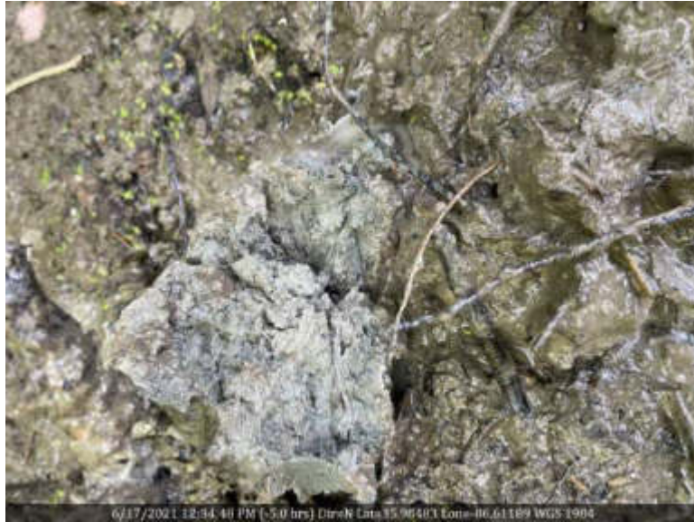
33 View of clay liner from upper portion of ISOPND-B, facing down.
