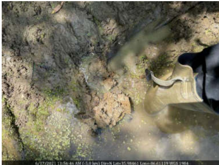
26 View of clay liner in ISOPND-A.
