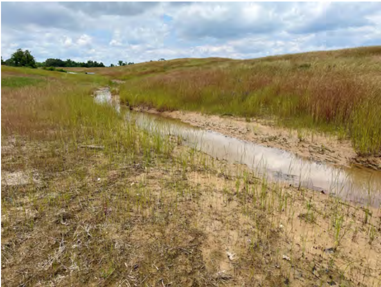
29 Stream 1-A Diversion, facing upstream and to the north
