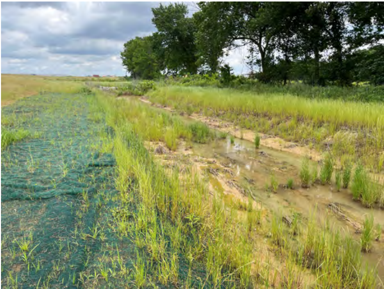
13 Stream 2 Diversion, looking upstream and to the east
