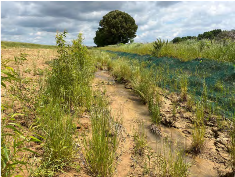
19 Stream 2 Diversion, looking upstream and to the east
