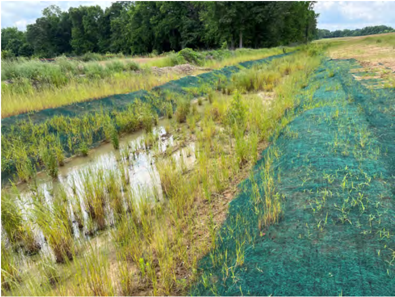
16 Stream 2 Diversion, looking downstream and to the west
