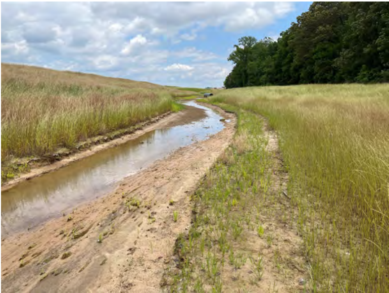
25 Stream 1-A Diversion, facing downstream and to the east
