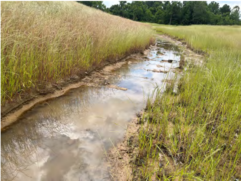
31 Stream 1-A Diversion SQT reach start location, looking downstream
