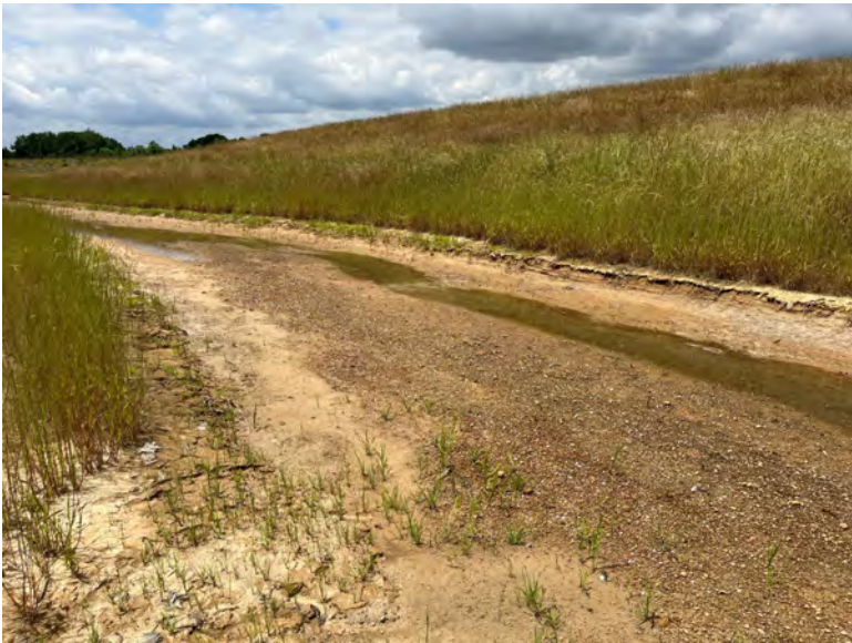
27 Stream 1-A Diversion, facing upstream and to the west
