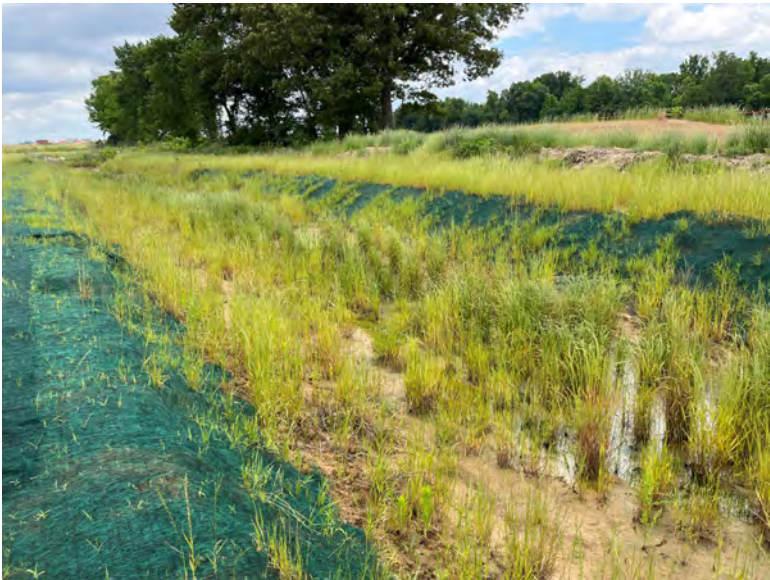
15 Stream 2 Diversion, looking upstream and to the east
