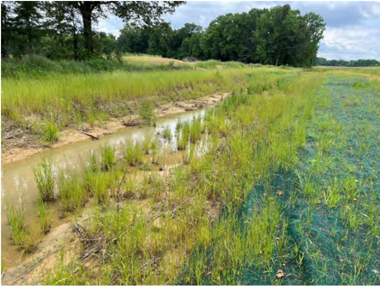
12 Stream 2 Diversion, looking downstream and to the west
