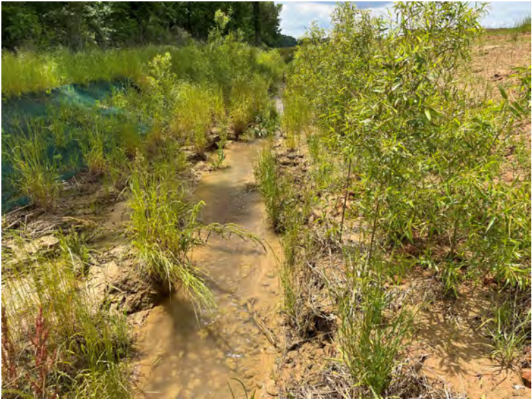
18 Stream 2 Diversion, looking downstream and to the west
