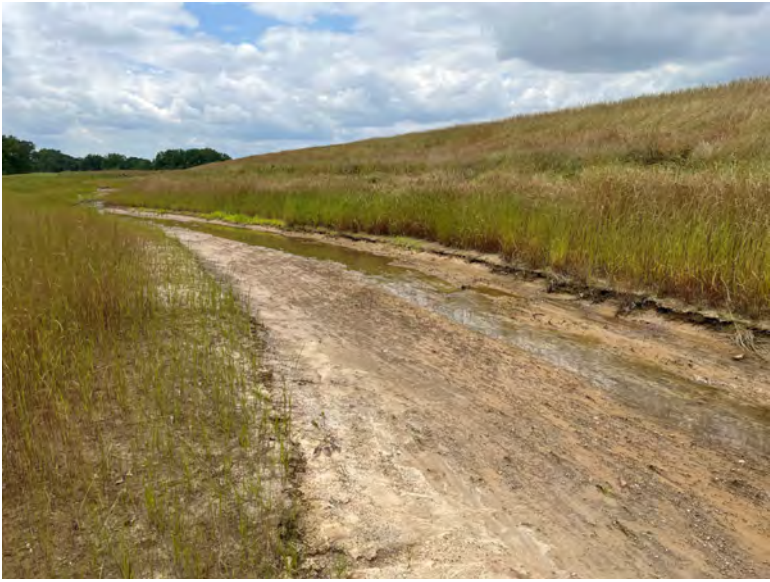
24 Stream 1-A Diversion, facing upstream and to the west
