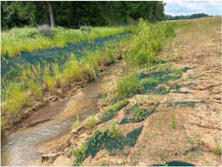
17 Stream 2 Diversion, looking downstream and to the west
