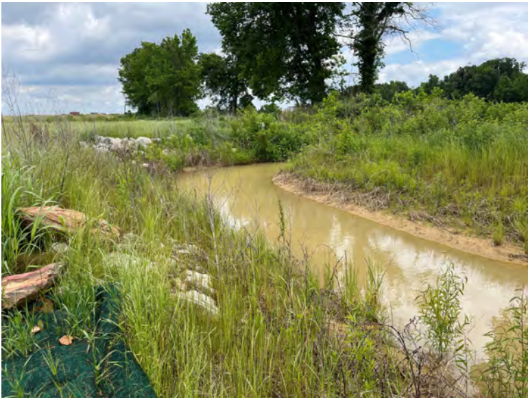
11 Stream 2 Diversion, looking upstream and to the east
