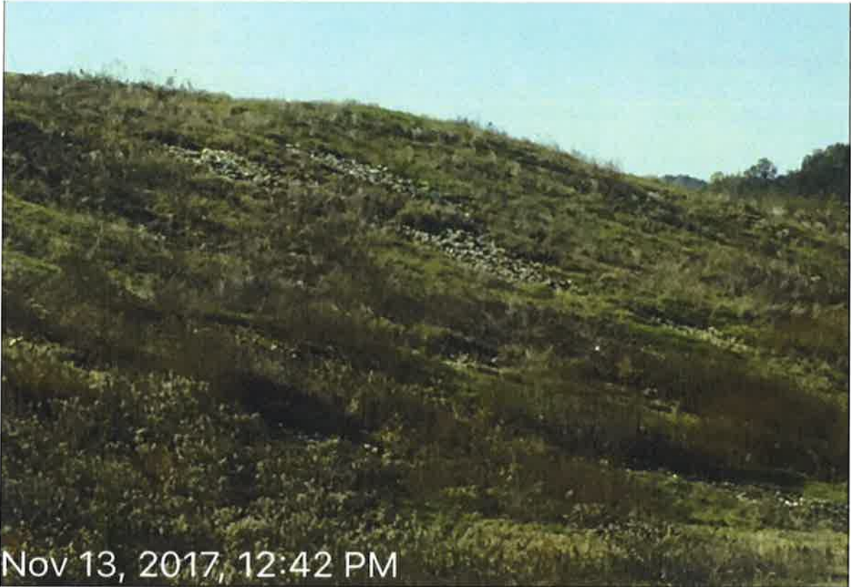
Picture 2. The City of Dyersburg Landfill inspection on November 13, 2017: Photo of unrepaired northern slope with erosion, washout of solid waste, unsatisfactory intermediate cover, and unsatisfactory stabilization of cover.
