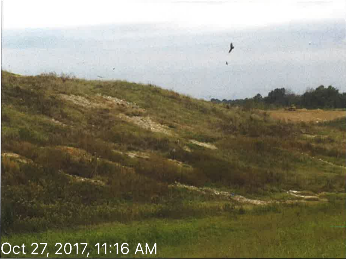
Picture 1. The City of Dyersburg Landfill inspection on October 27, 2017: Photo of northern slope with erosion, washout of solid waste, unsatisfactory intermediate cover, and unsatisfactory stabilization of cover.
