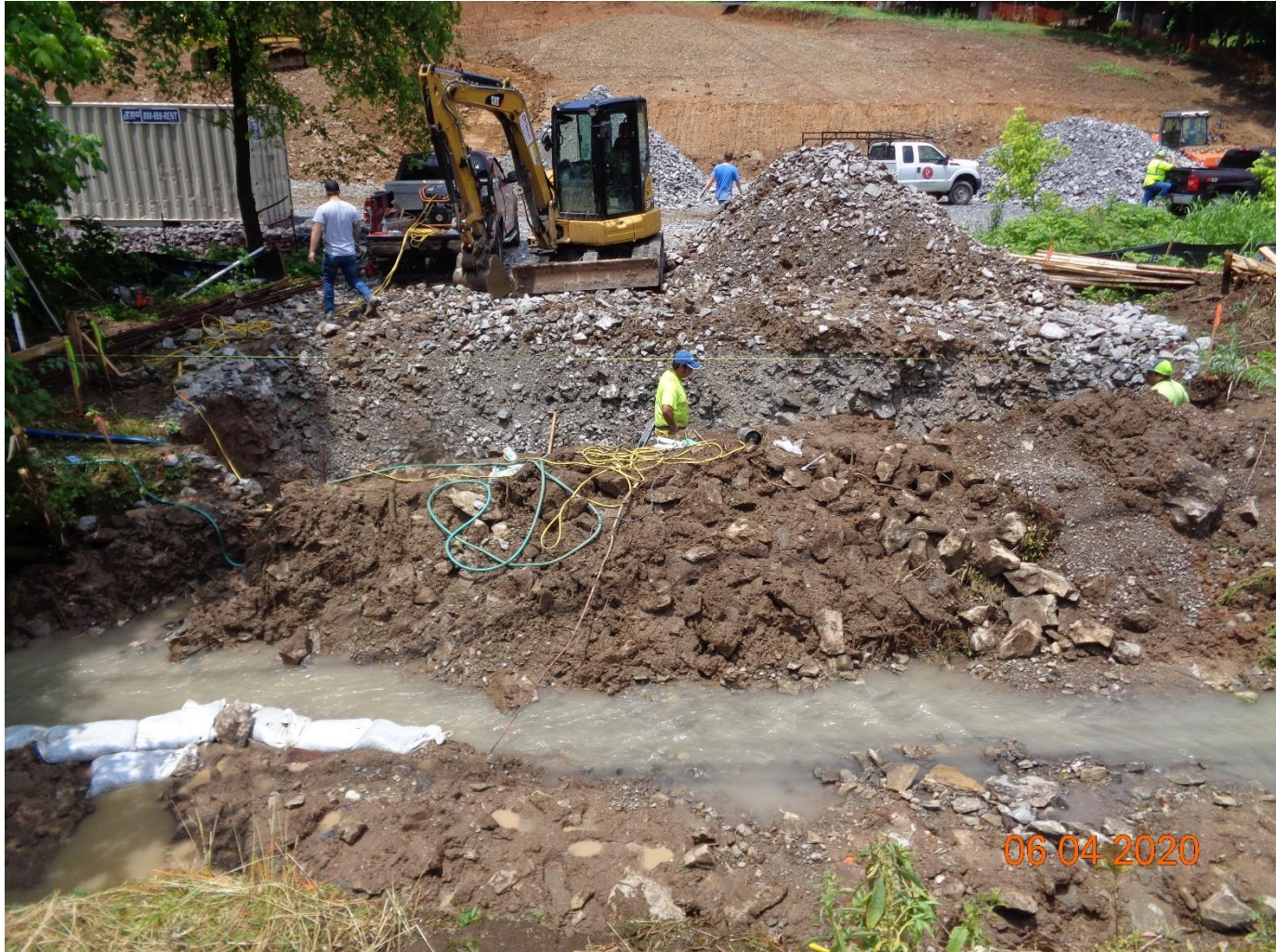
Photo 5: View of ARAP NRS16.124 construction area.
