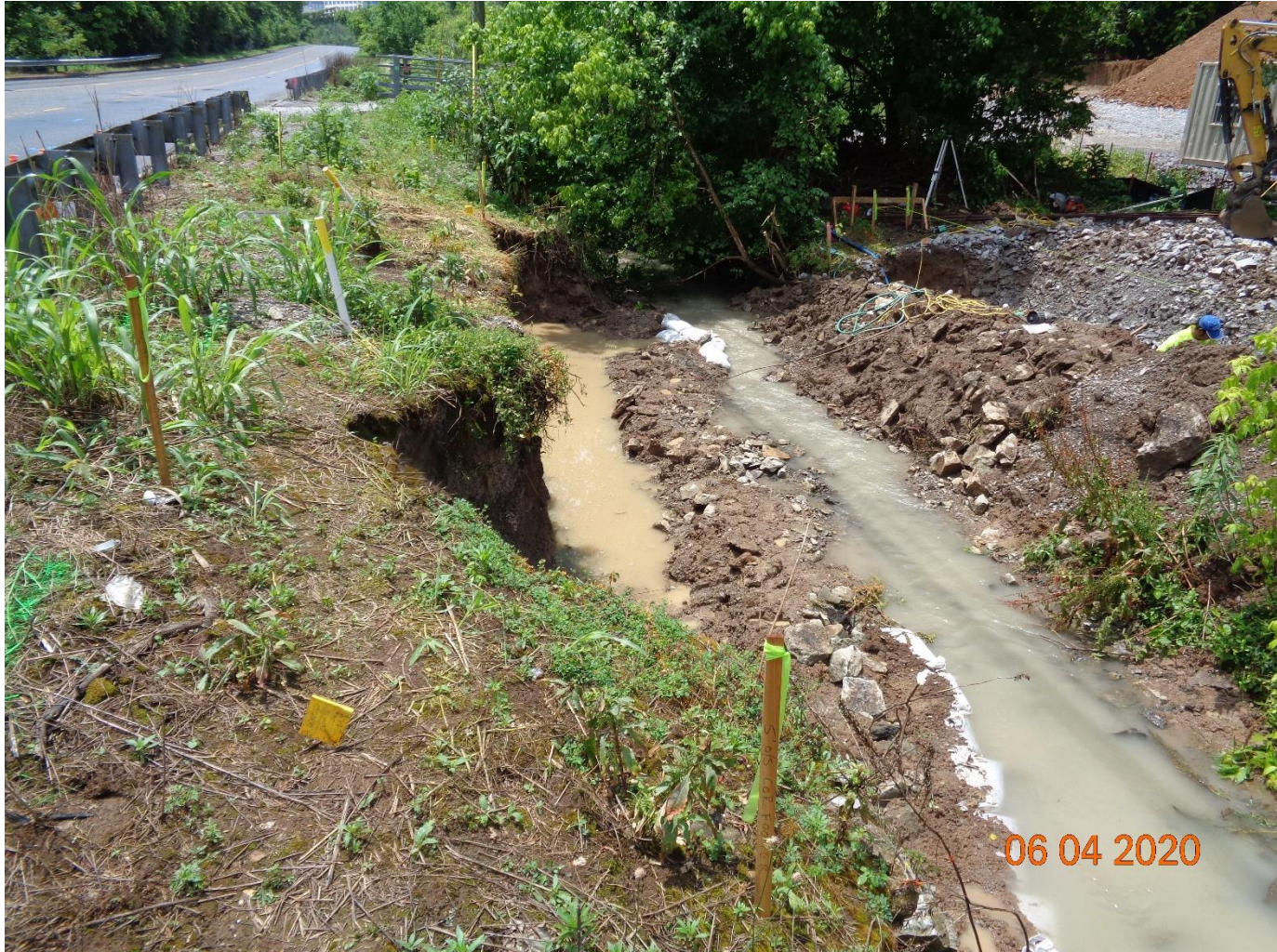
Photo 4: View of ARAP NRS16.124 construction area looking south.
