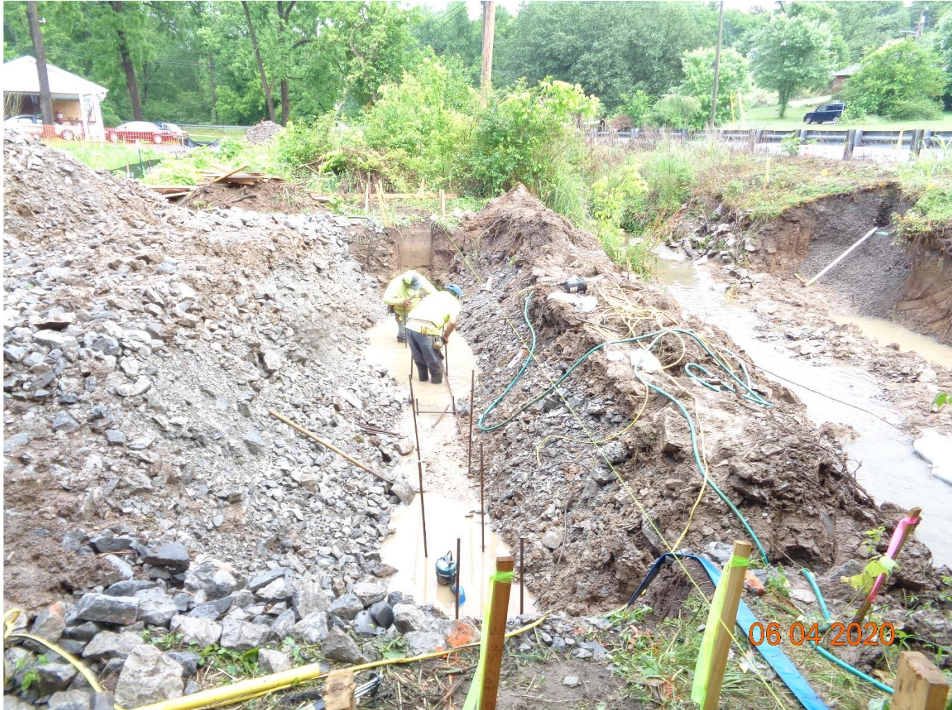
Photo 2: View of ARAP NRS16.124 construction area.
