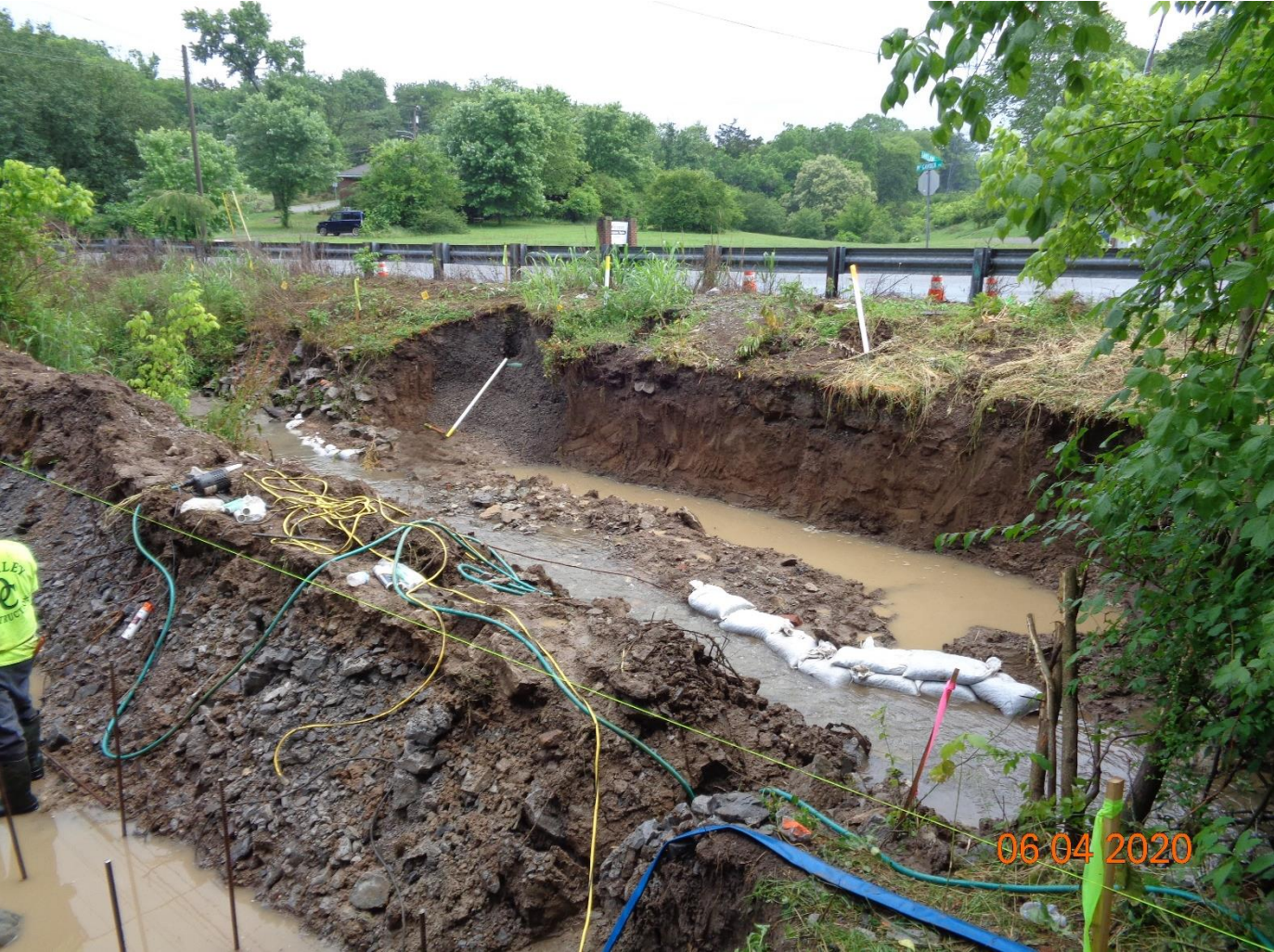
Photo 3: View of NRS16.124 construction area.
