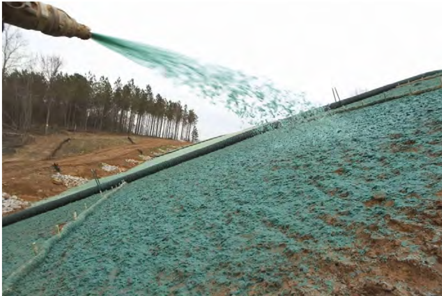
Hydraulically applied seed, mulch and binder
