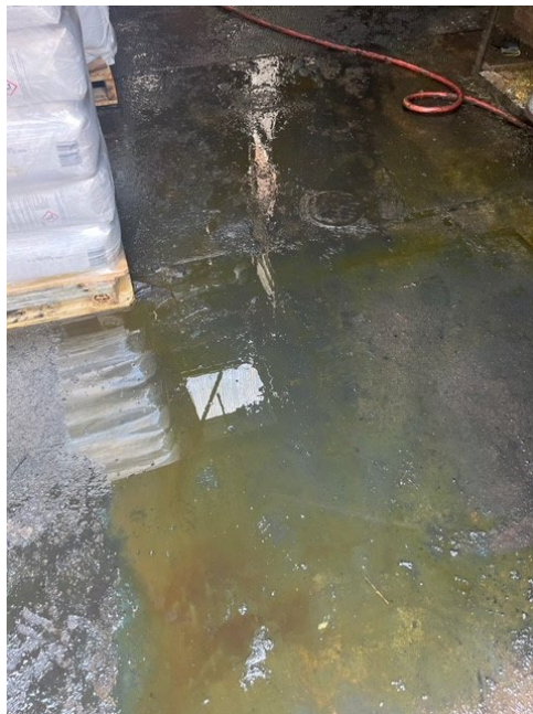
Figure 3. (Oil Overflow at Used Oil Tank)
