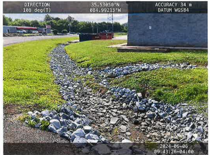
Photo 6: Rip rap swale to Outfall 001.
