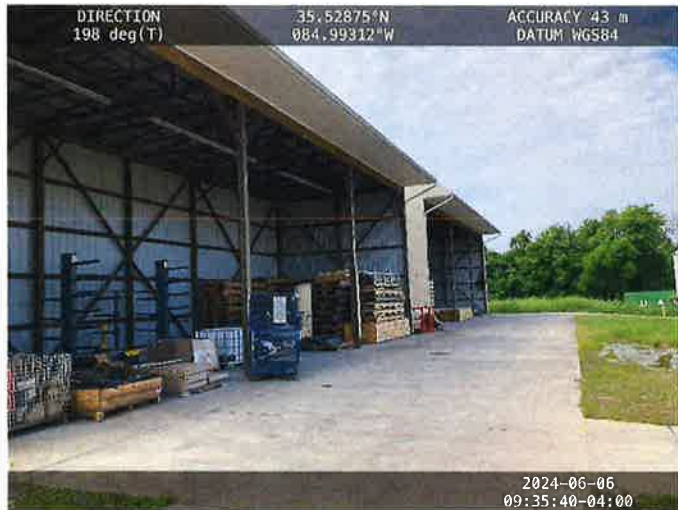
Photo 3: Covered storage near south loading area.
