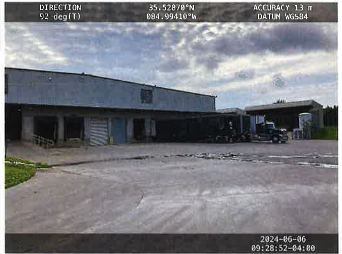
Photo 2: South lot of facility; loading zone.
