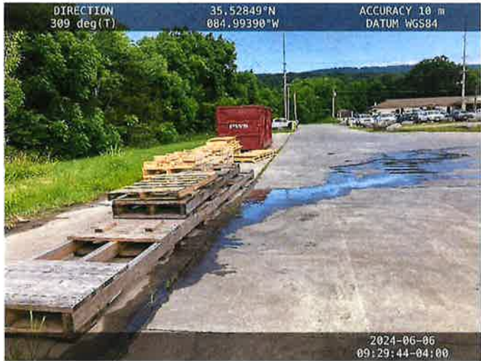
Photo 5: South lot drainage just above Outfall 002.
