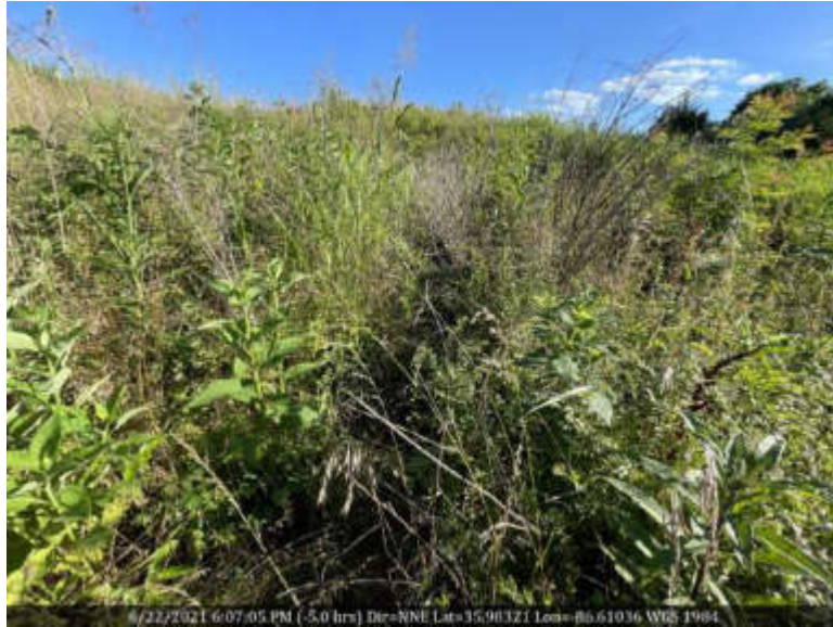
11 View of D-2 upper reach, facing upslope/southwest along detention pond embankment.
