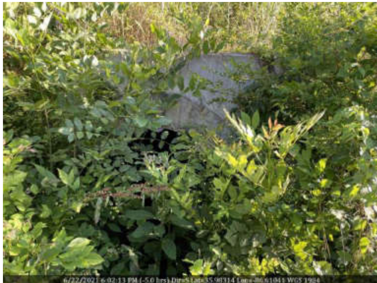
12 View of detention pond outlet culvert, facing upslope/southwest.
