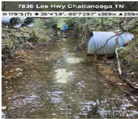
Photo 3: HD 1 ( Friar Branch) flowing water in Channel after 7 days with no significant rain event.
