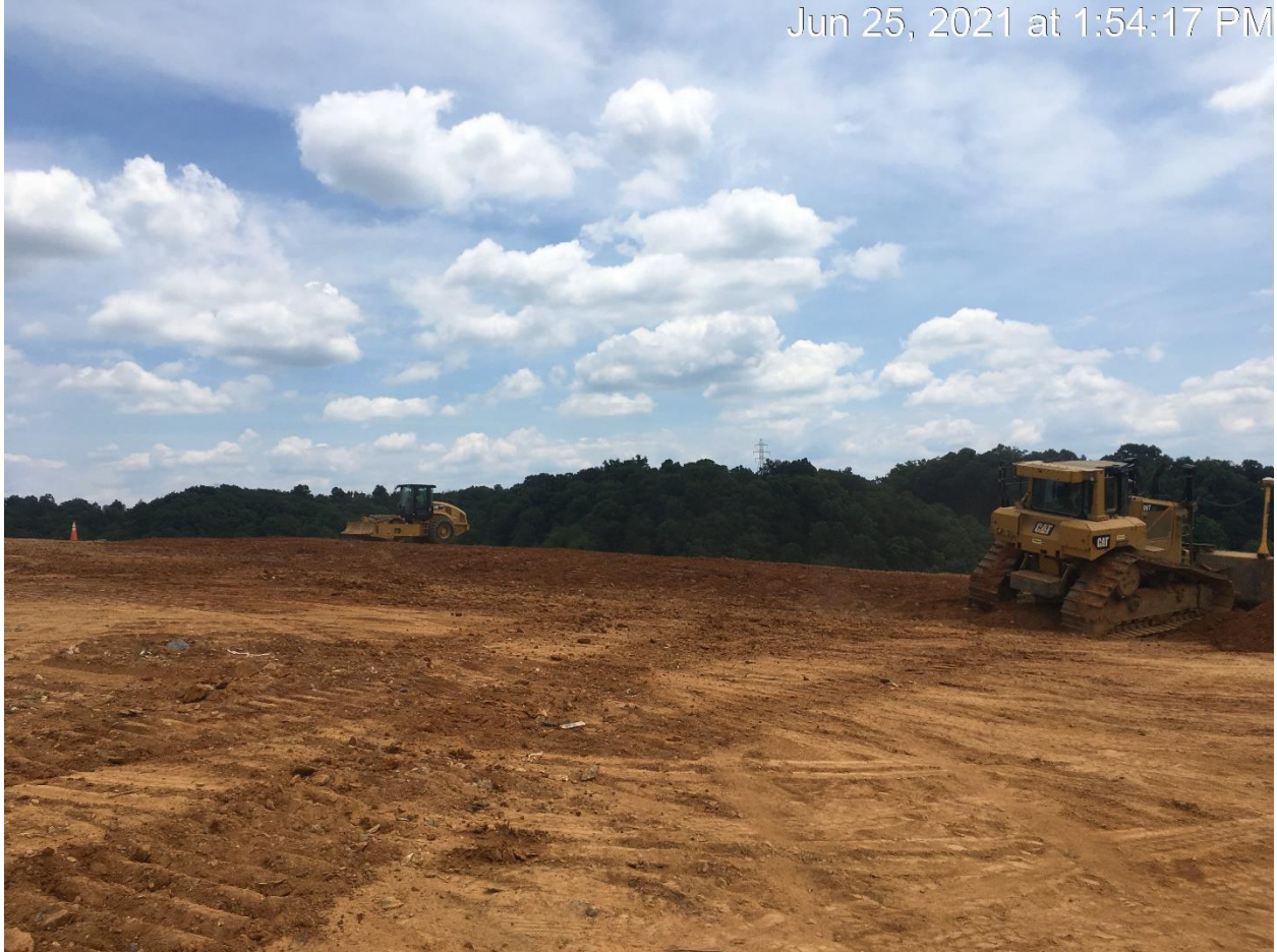
Figure 2: EDGE OF CLAY LINER INSTALLED
