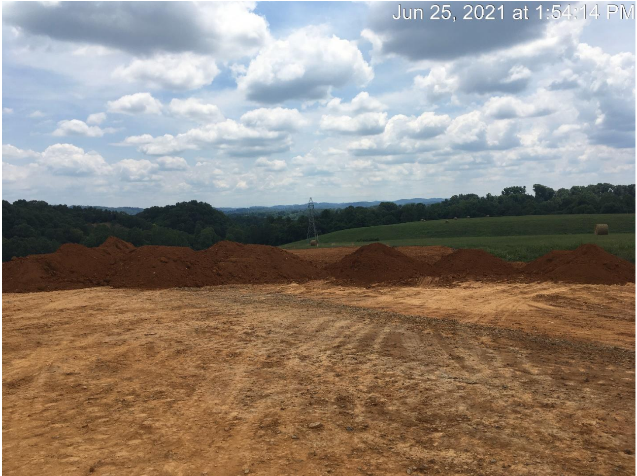
Figure 1: CLAY BEING HAULED INTO THE SITE
