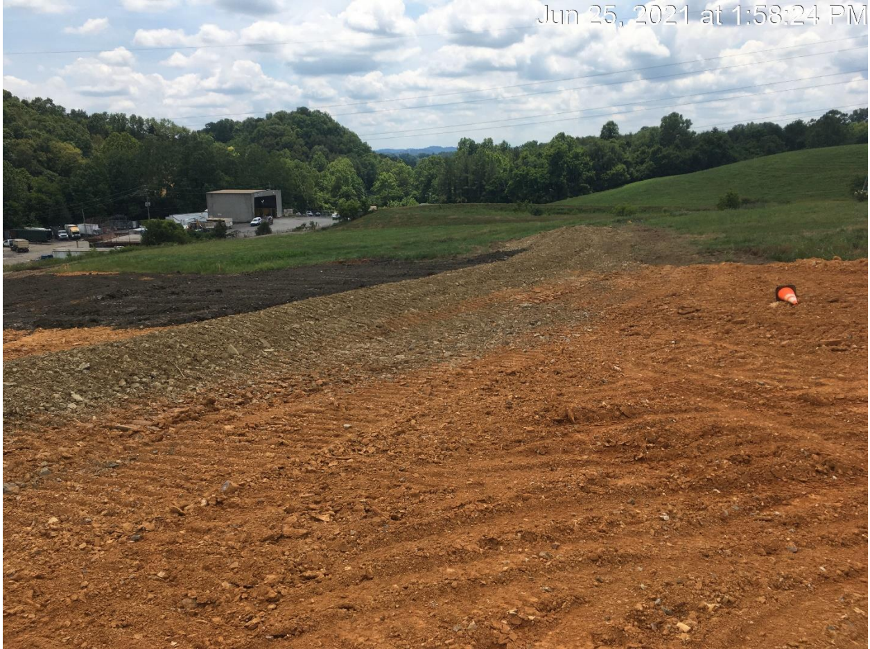
Figure 5: TACK-ON BERM CONSTRUCTED OF SHALE OVER THE CLAY LINER
