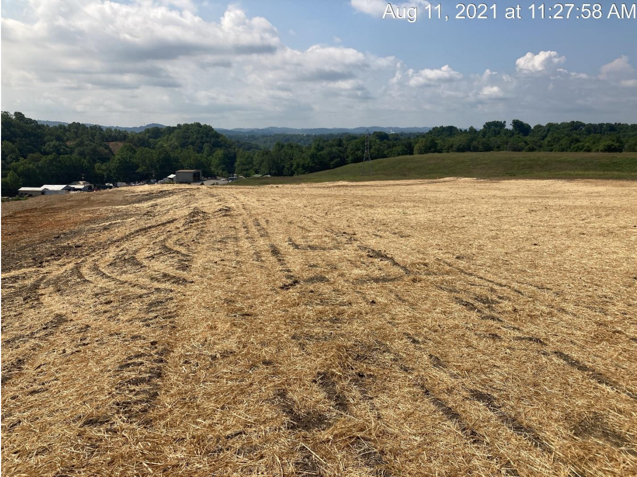
Figure 13: EASTERN EDGE OF THE CLOSURE AREA ( LOOKING SOUTH)
