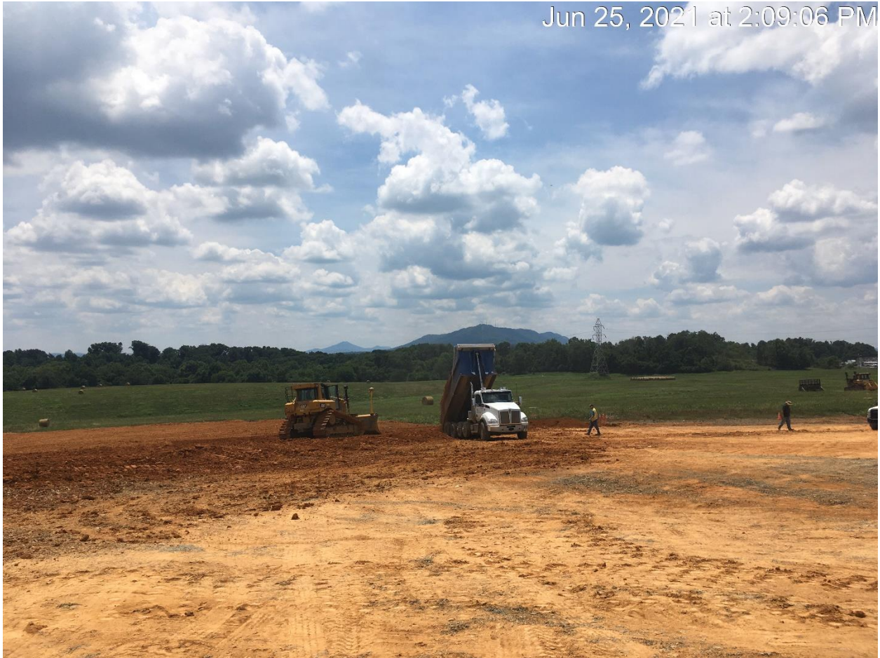
Figure 12: EDGE OF CLAY LINER CONSTRUCTED TO-DATE
