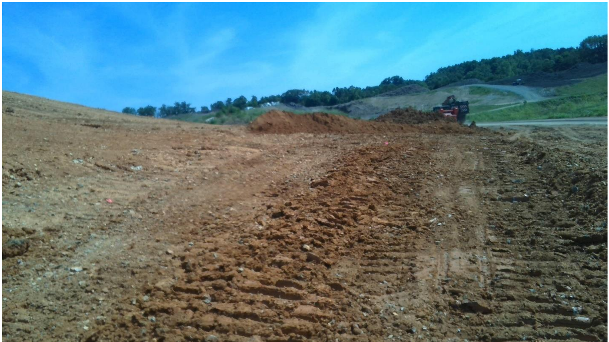
Photo 8: Connection Trench after Backfilling and Compacting with Track Loader
