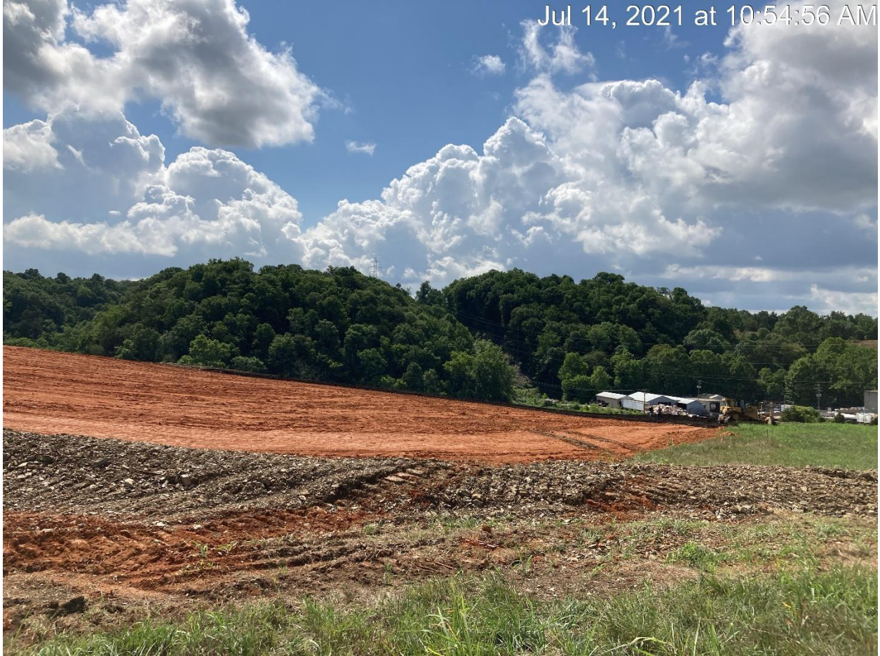
Figure 1: 3RD TACK-ON BERM INSTALLED
