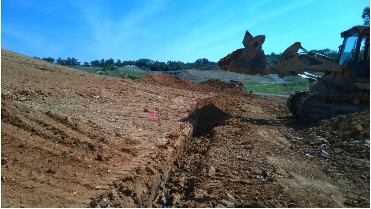
Photo 7: Track Loader Backfilling the Connection Trench with Clay
