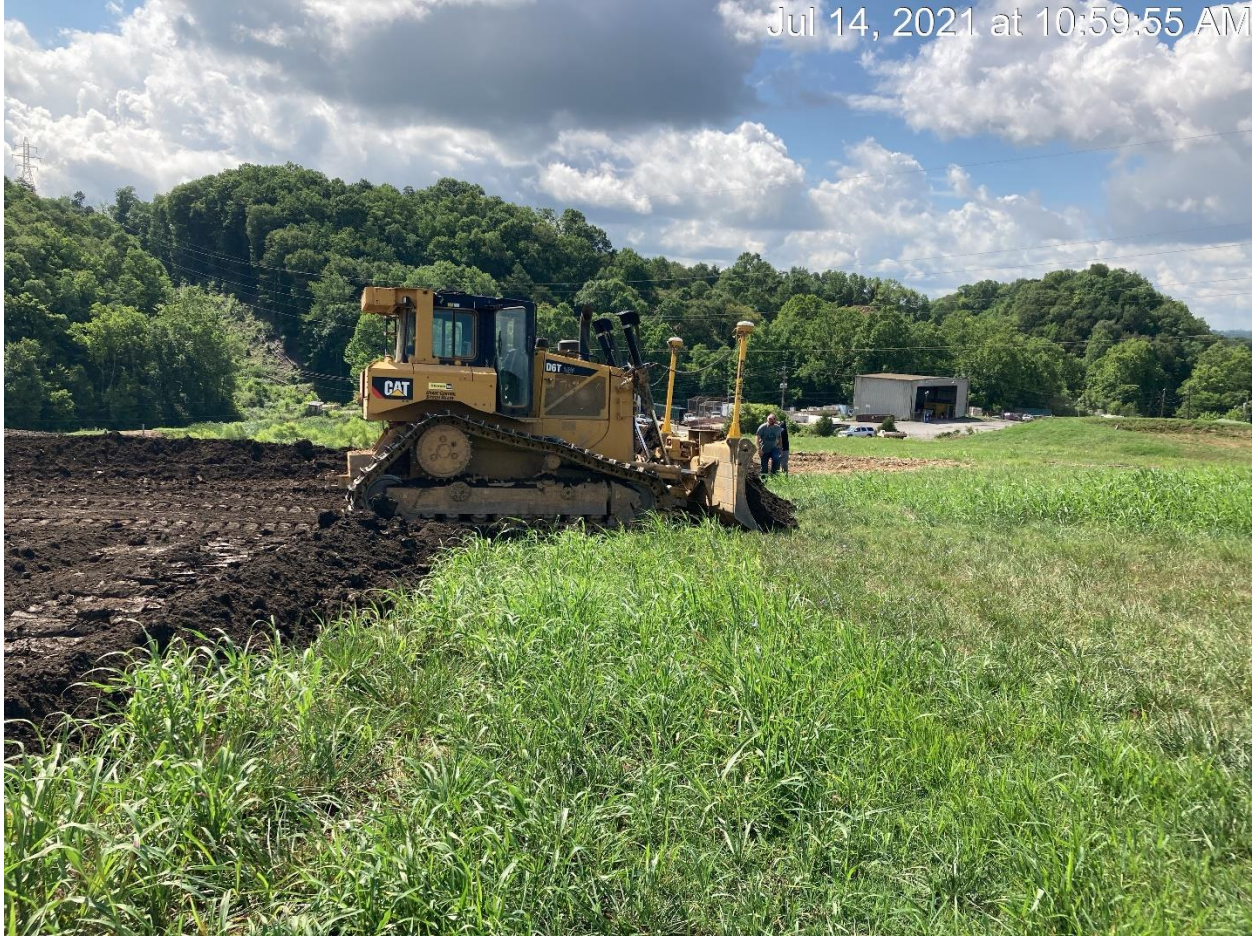
Figure 5: CLOSER LOOK AT THE TOPSOIL
