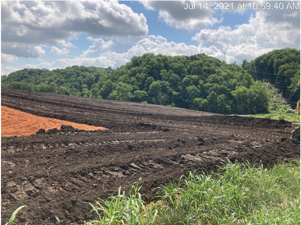
Figure 4: INSTALLATION OF THE TOPSOIL BETWEEN THE 1ST AND 2ND TACK-ON BERM
