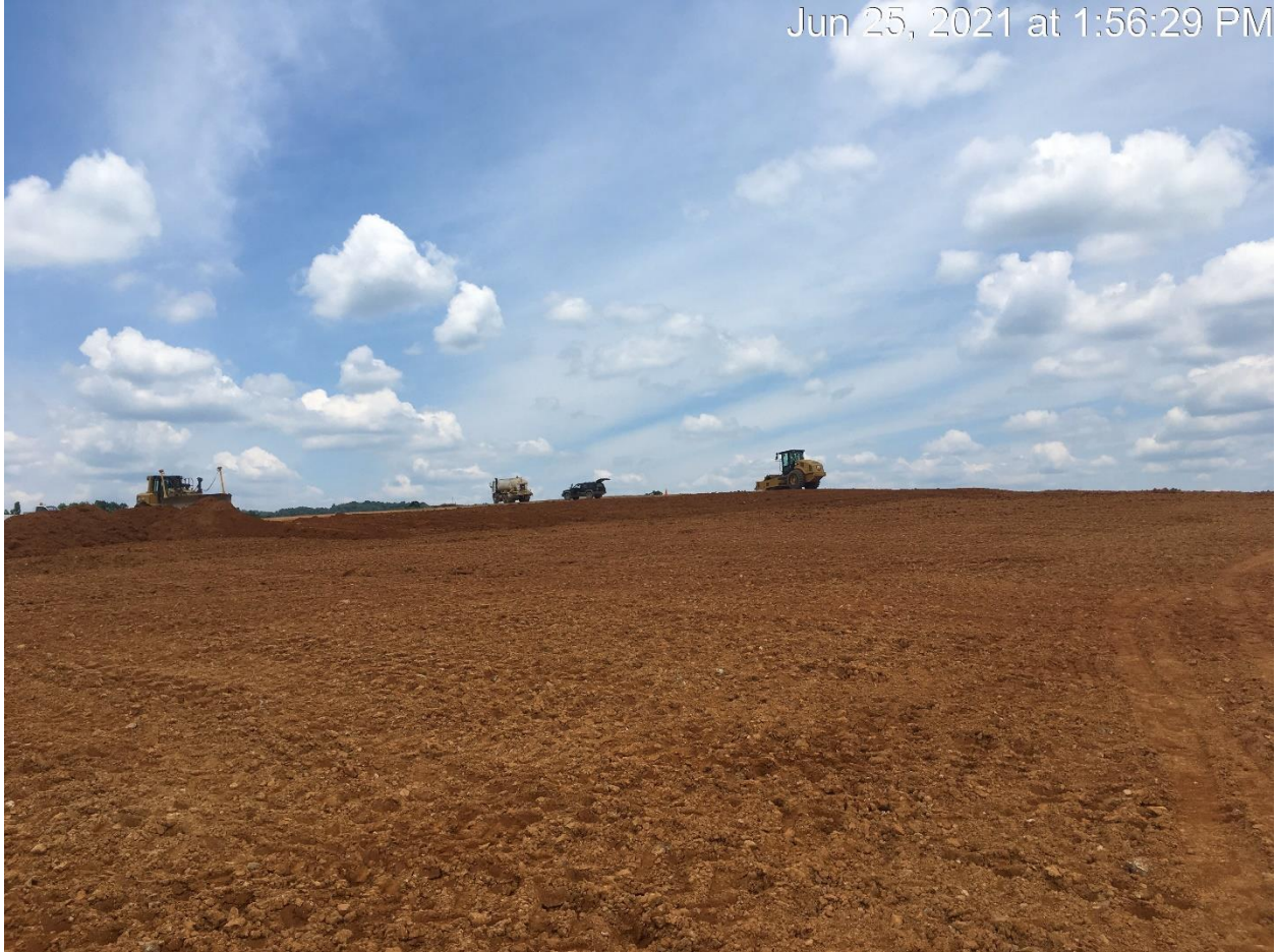
Figure 3: CLAY LINER BEING COMPACTED
