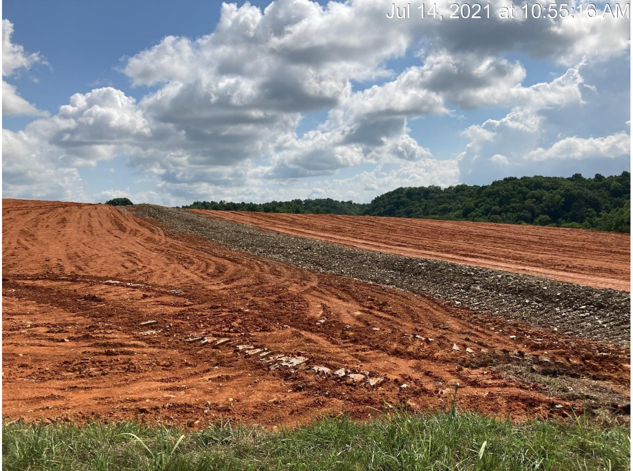
Figure 3: 2ND TACK-ON BERM
