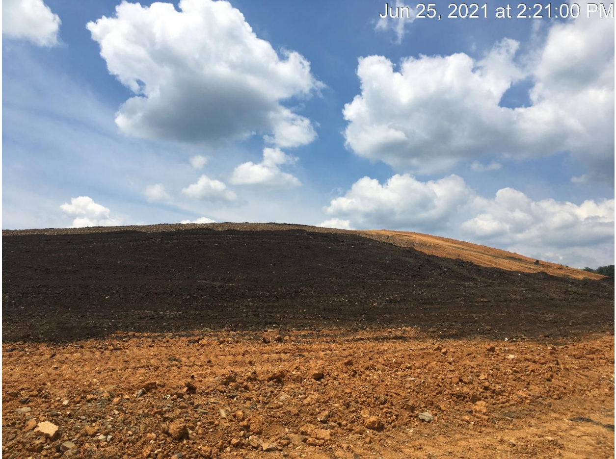
Figure 13: EASTERN SLOPE WITH TOPSOIL INSTALLED
