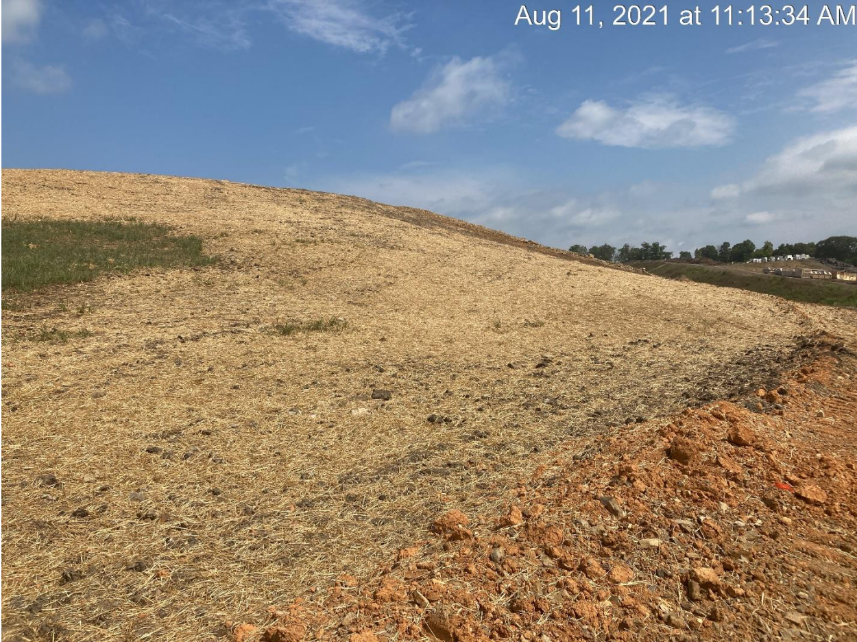
Figure 2: SOUTHERN END OF THE CLOSURE AREA (EAST SIDE)
