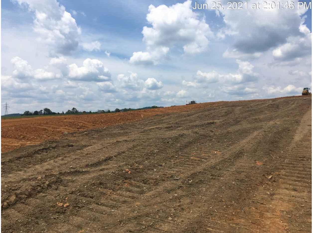
Figure 10: NORTHERN EDGE OF CLAY LINER
