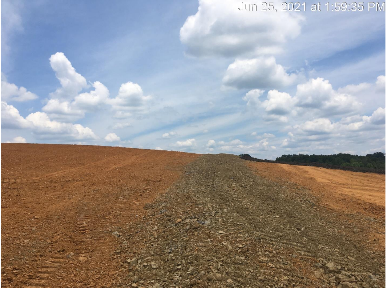
Figure 8: SECOND TACK-ON BERM ( LOOKING NORTH)
