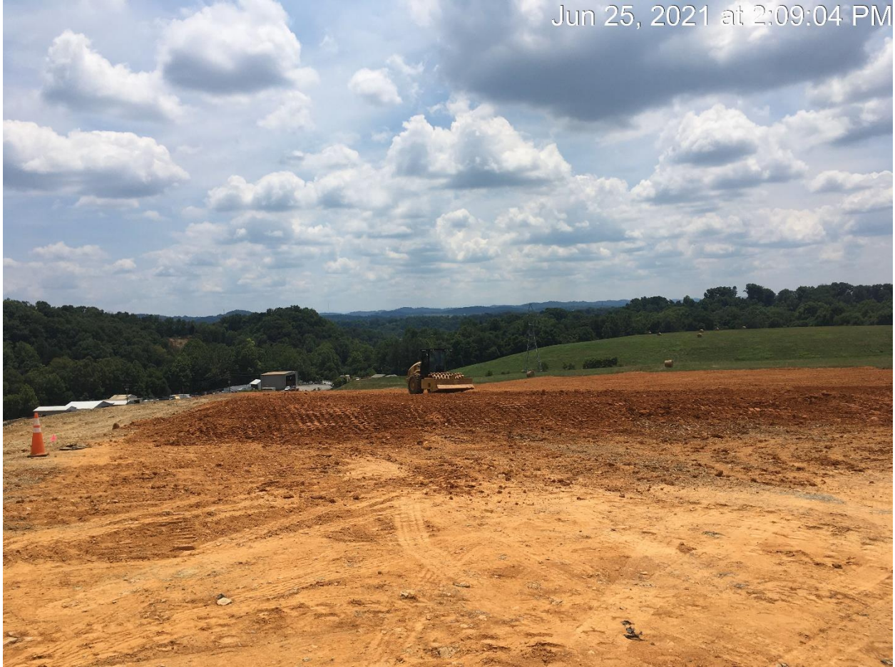
Figure 11: EDGE OF CLAY LINER OF WHAT HAS BEEN CONSTRUCTED
