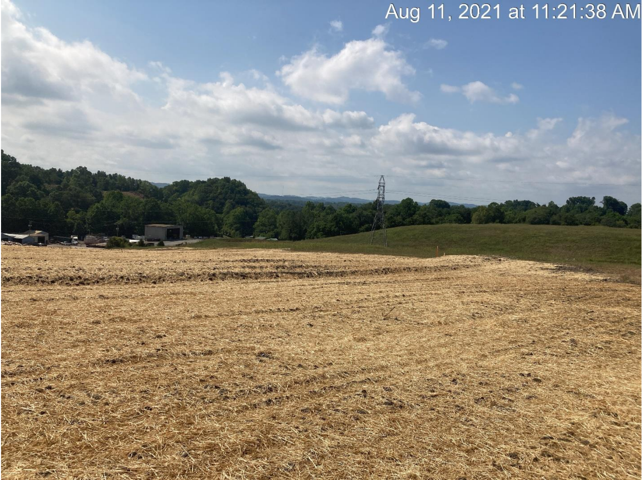
Figure 5: DRAINAGE BERM (LOOKING WEST)
