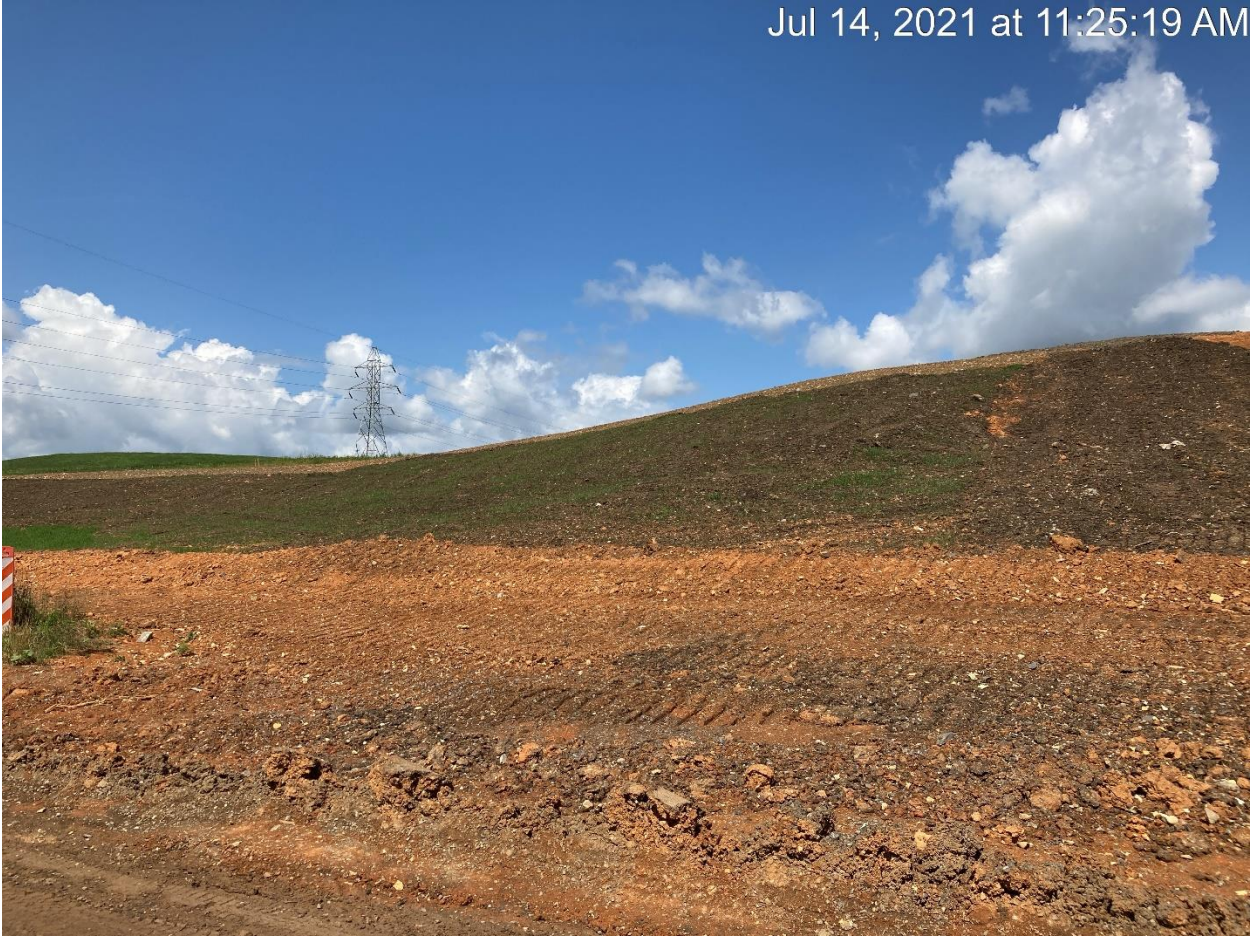
Figure 7: EASTERN SLOPE TOPSOIL GROWING GRASS
