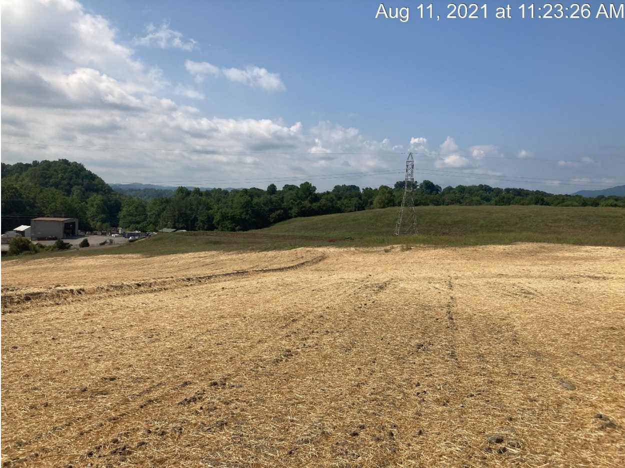
Figure 8: SECOND DRAINAGE BERM
