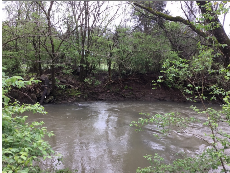
Photo 10 - View of Erosion Site
