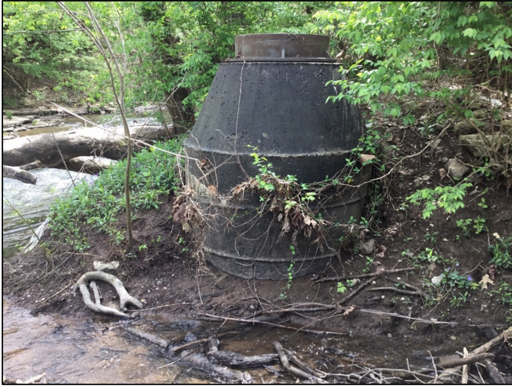
Photo 4 - View of Exposed Pipe (Manhole)
