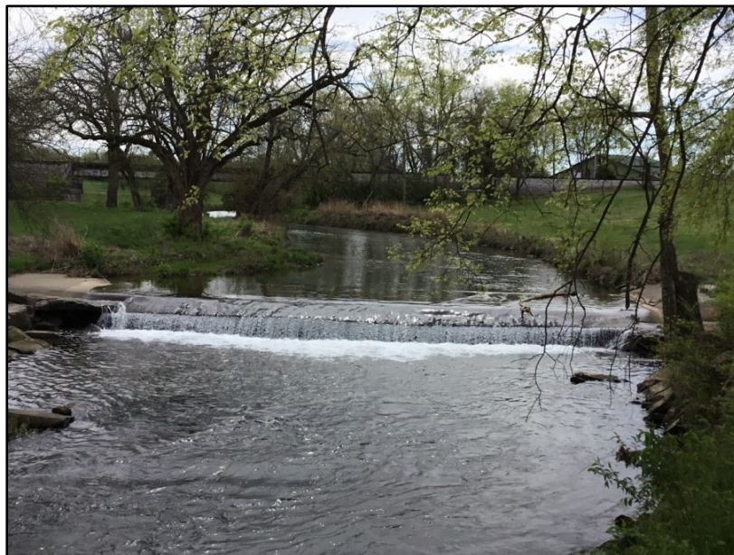
Photo 6 - View of the Fish Barrier
