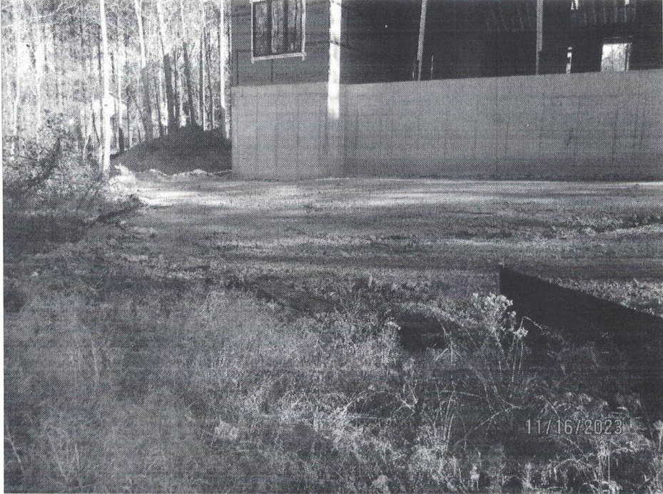
Photo 5: Outfall S208 Silt Fence has fallen over and needs repair. Photo Taken 11/16/2023
