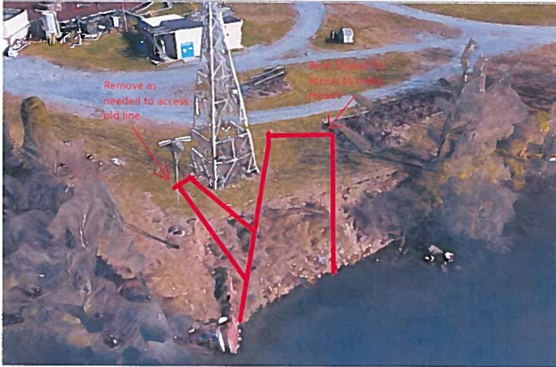
Photo 3: North Bank of River
