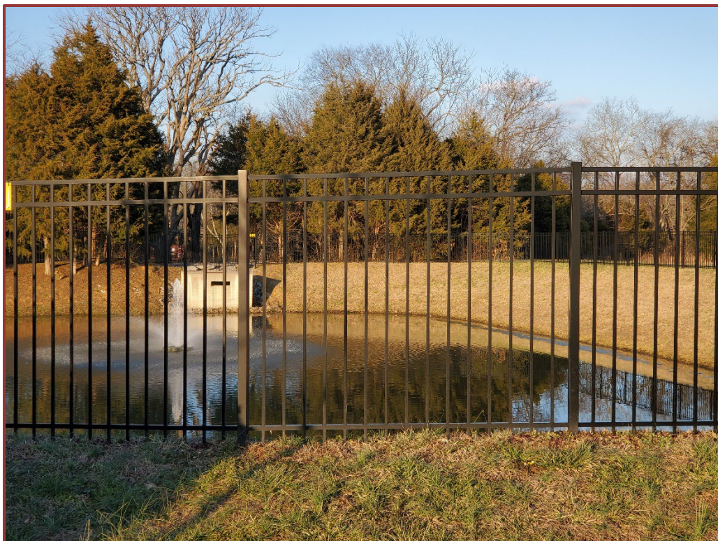
View of Pond and Outfall Structure - Phases 7, 8, and 9
