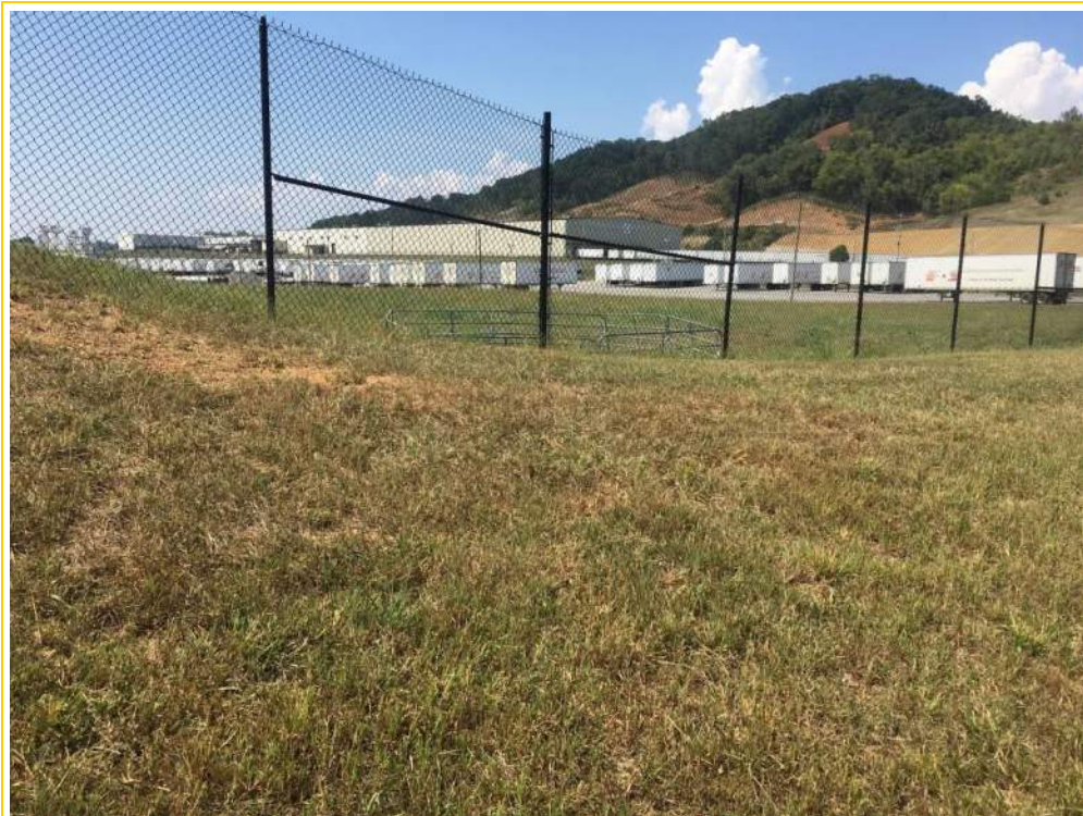
Photo 4 – General view of the outlet junction box, looking north towards the existing truck parking area where pipe replacement is proposed.
