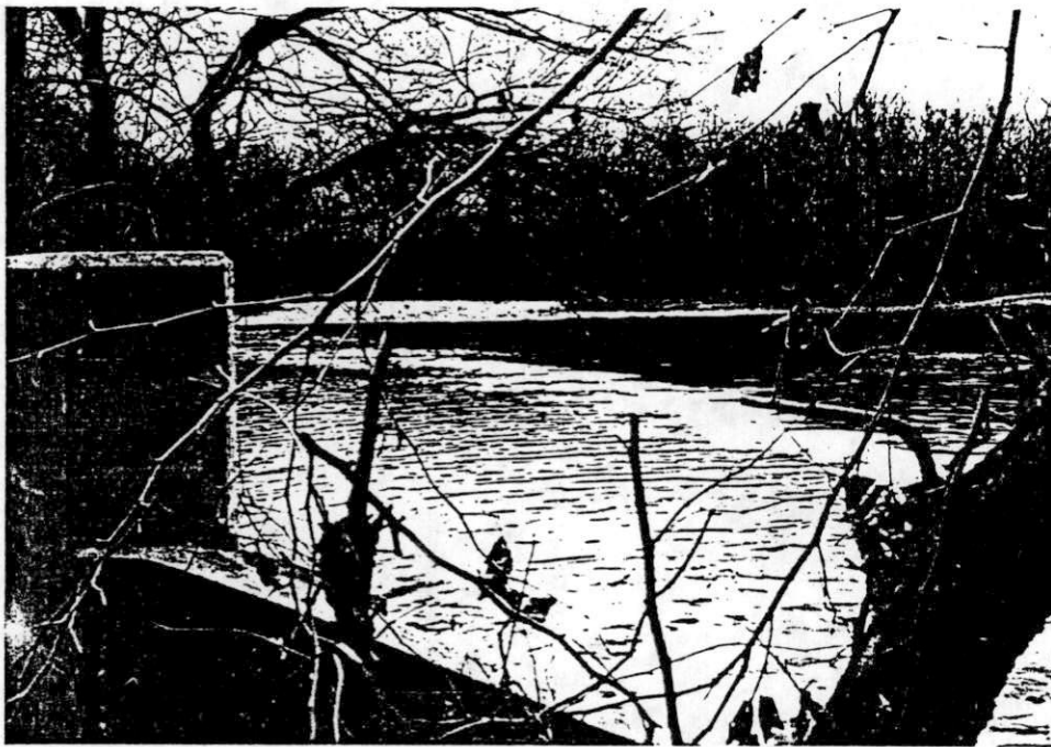
A-13. Slightly downstream of current NUB discharge (low water level)
