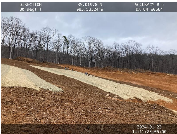
Photo 11: Matting currently being installed along slope above basin.
