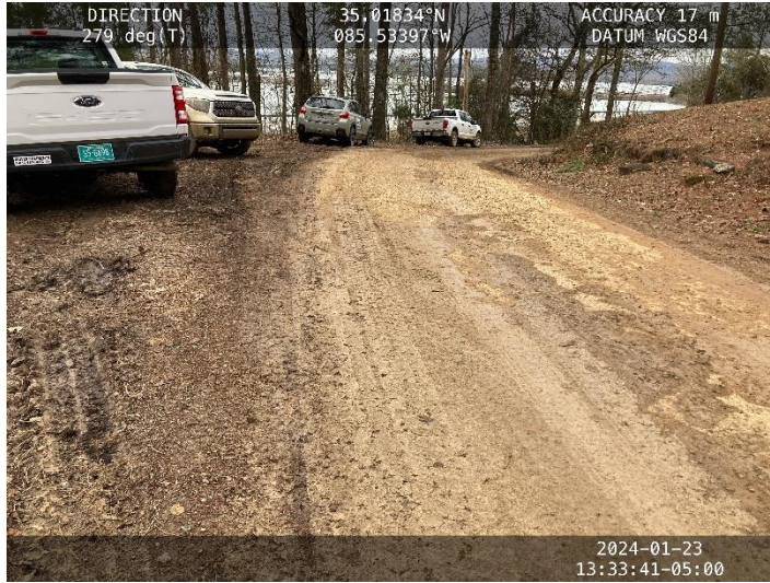
Photo 1: Track out along Whiteside Loop.
