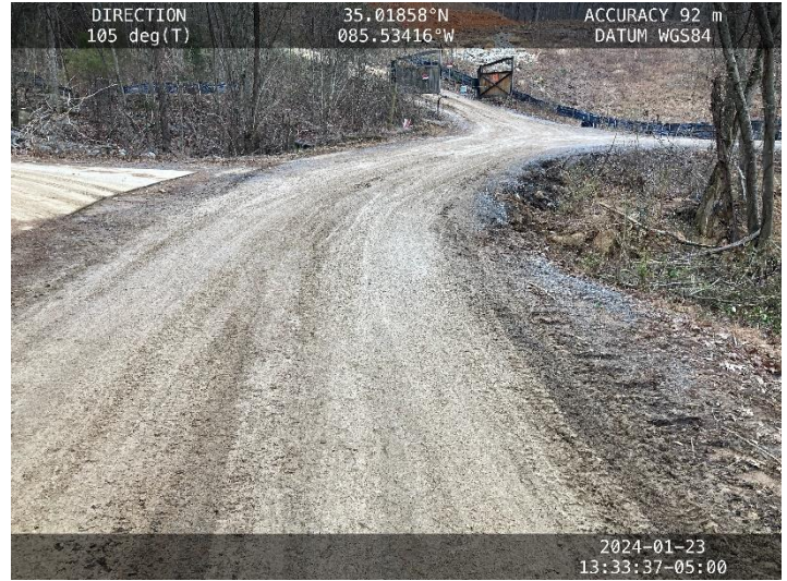
Photo 2: Facing site entrance from Whiteside Loop.
