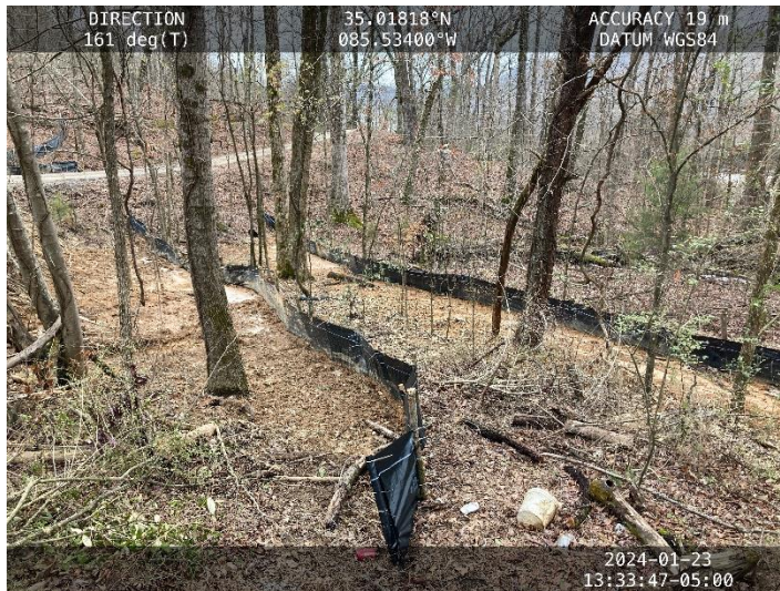
Photo 3: Off site sediment in wet weather conveyance just below Photo 2. Flows to reservoir.
