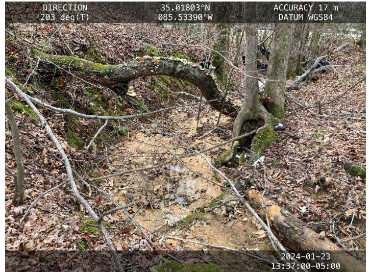
Photo 6: Evidence of off site sediment accumulation in WWC.
