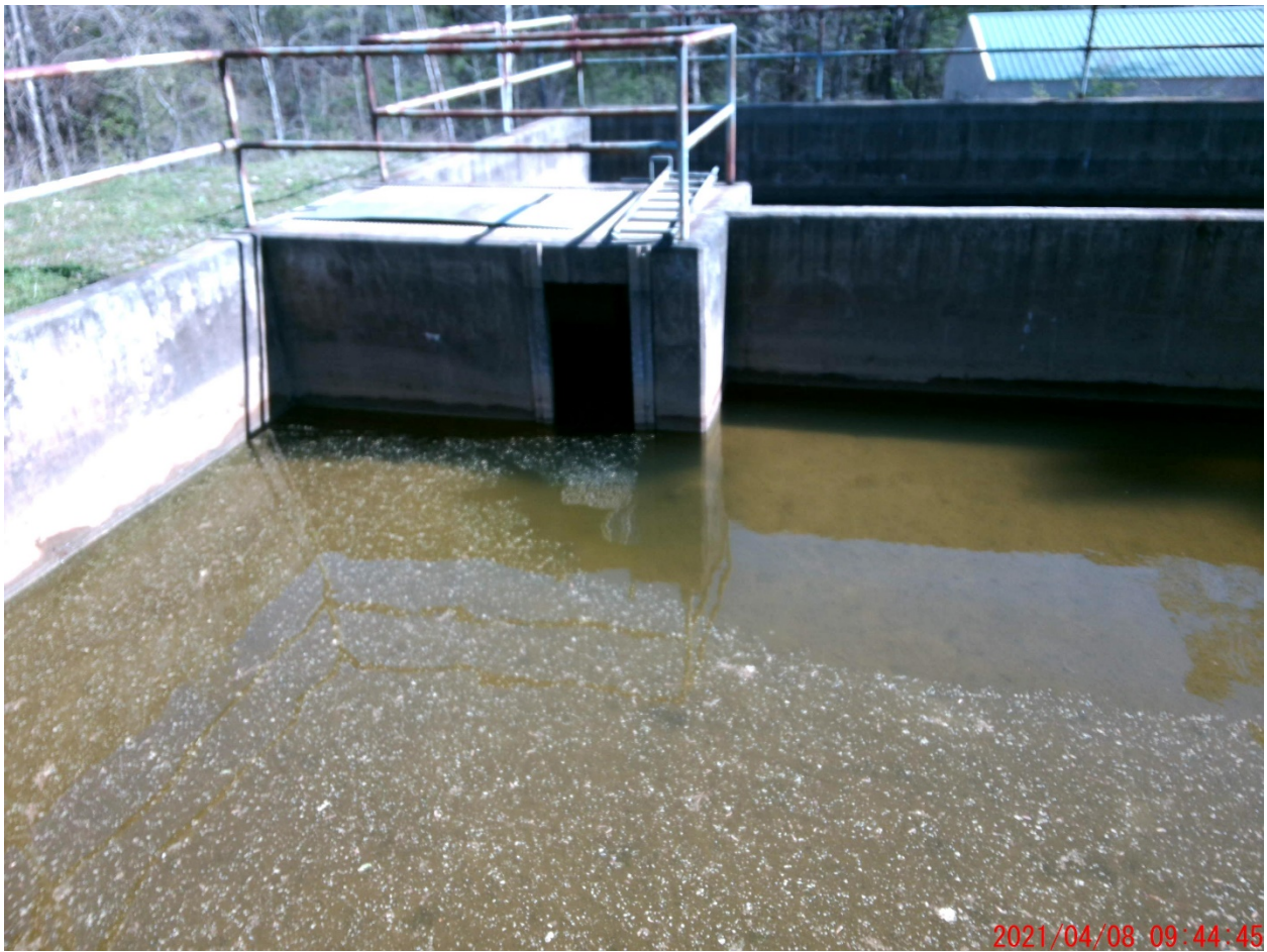
Image 2 - Sedimentation Basin Splitter at Influent
