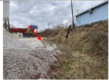
Looking Northeast along Old Jacksboro Rd. Any stormwater that comes off the road is collected along a channel that goes to Hunter Branch. The next photo shows a ditch to another Outfall point that should be added to Stormwater monitoring plan as 003 since it goes to Hunter Branch.
