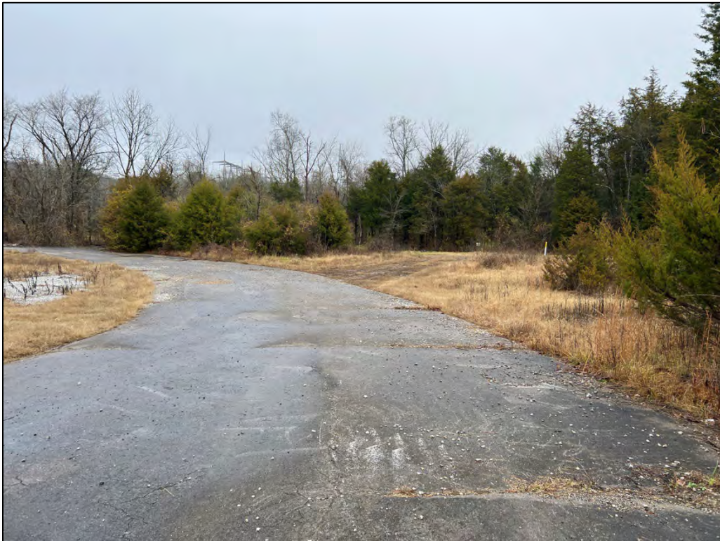
Photograph pp01 view North
