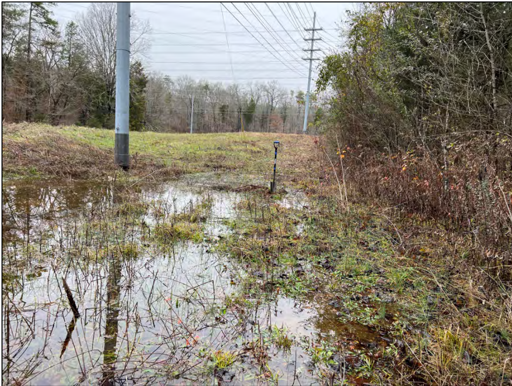
Photograph pp47 view North
