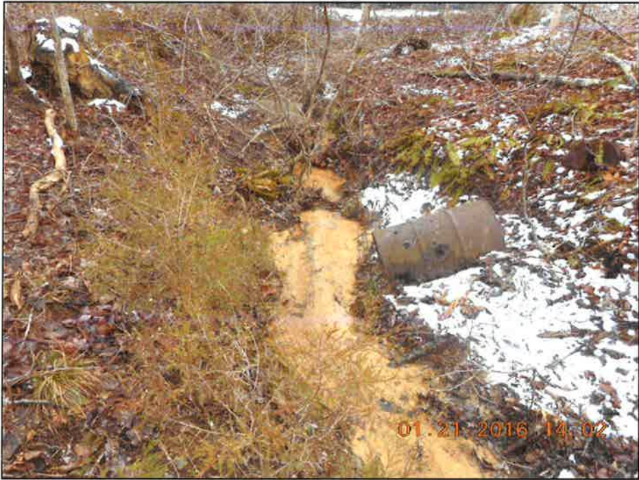
Photo 4: Stream channel filled with sediment immediately below the crossing.
