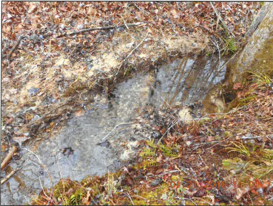
Photo 3: A section of the tributary immediately upstream of the crossing.
