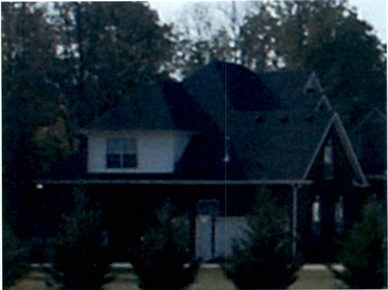
Home at Royal Glenn – Consolidated Utility District, Rutherford County, TN
