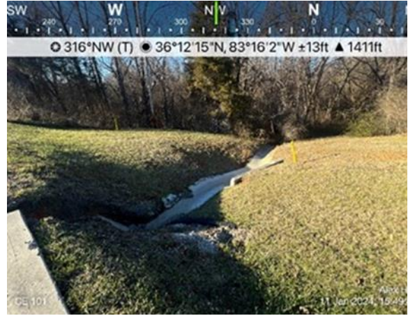
Photo 10: Representative view of vegetative restoration/stabilization at WWC 7.
