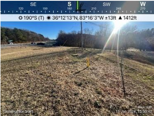
Photo 11: Representative view of vegetative restoration/stabilization at Construction Exit #1.
