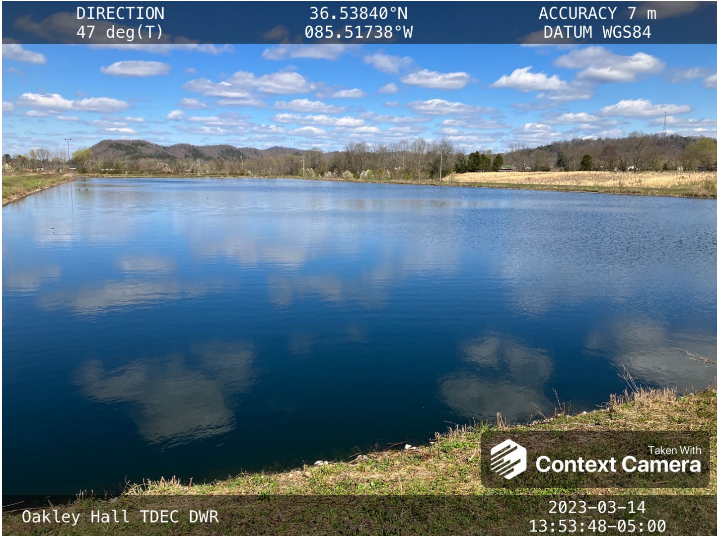
The third lagoon of the three in the series is pictured. Various wild birds were using the lagoon. Algae was present in the water column. This lagoon is to be inspected for sludge/solids depth.
