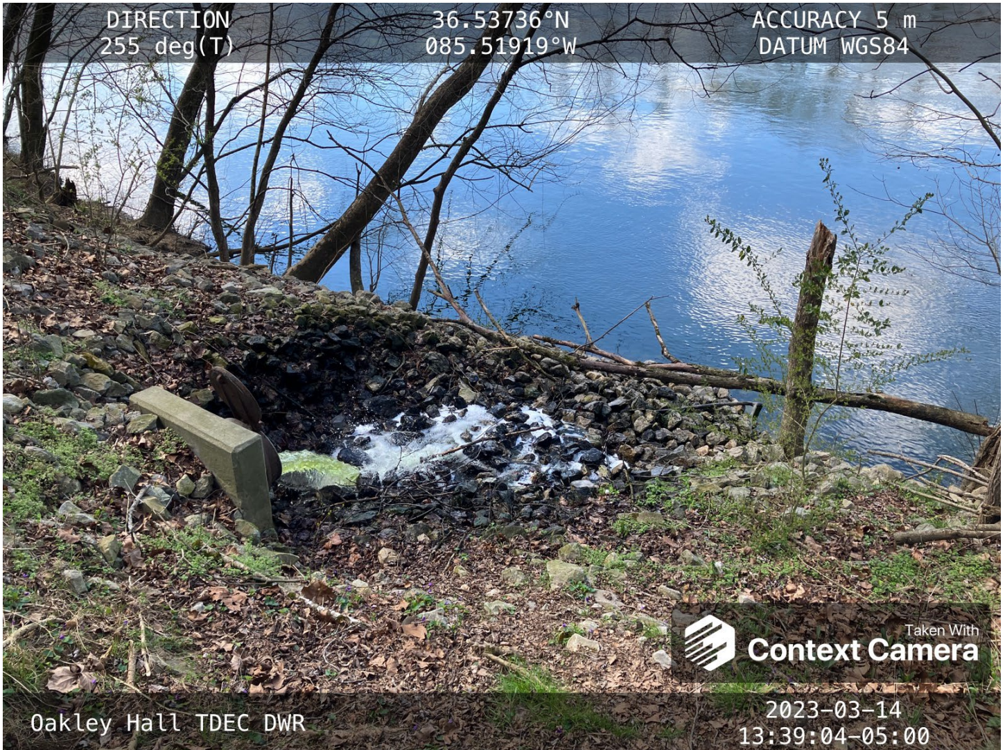
The effluent outfall is pictured. It is entering the Cumberland River. A color contrast was not observed in the river. Foam was not present in the outfall into the Cumberland River.
