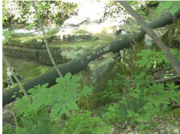
Photos showing debris around pipe, a tap, rock pipe supports, and complete separation of pipe.
