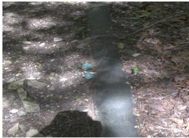
Photos of surface routing and taps towards to the top of the mountain. Bays Mountain Road can be seen at the top of one of the photos.
