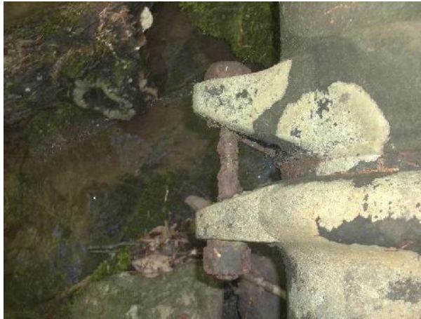
Photos of surface crack along pipe, stone enveloping pipe support, and severe corrosion of bolt.
