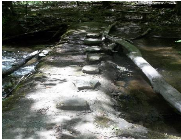
First crossing of abandoned water line across Dolan Branch in Eastman Chemical Company property as well as an abandoned gate valve
