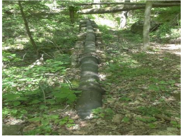
Photos showing fracture in pipe as well as rock pile pipe support and surface routing of abandoned line
