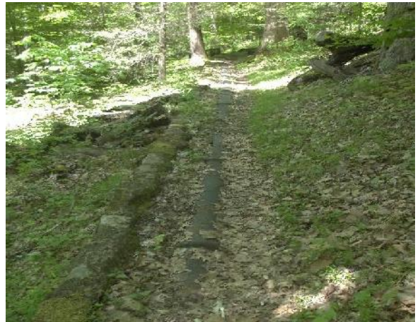
Photos showing rock pipe support and general surface routing of pipe
