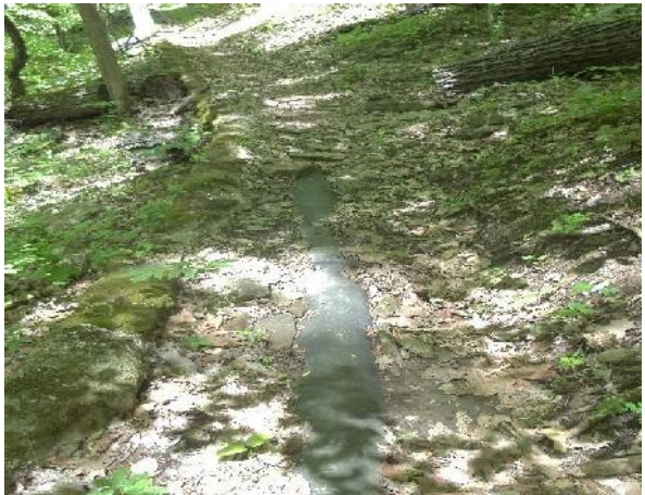
Photos showing rock pipe support and general surface routing of pipe
