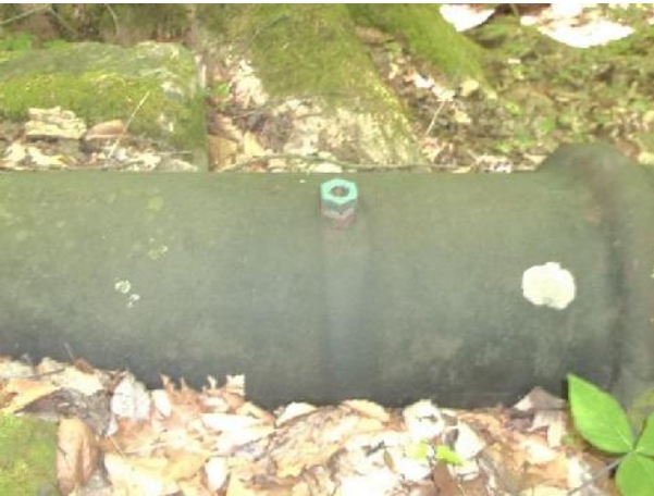
Depictions surface routing and taps in old water line
