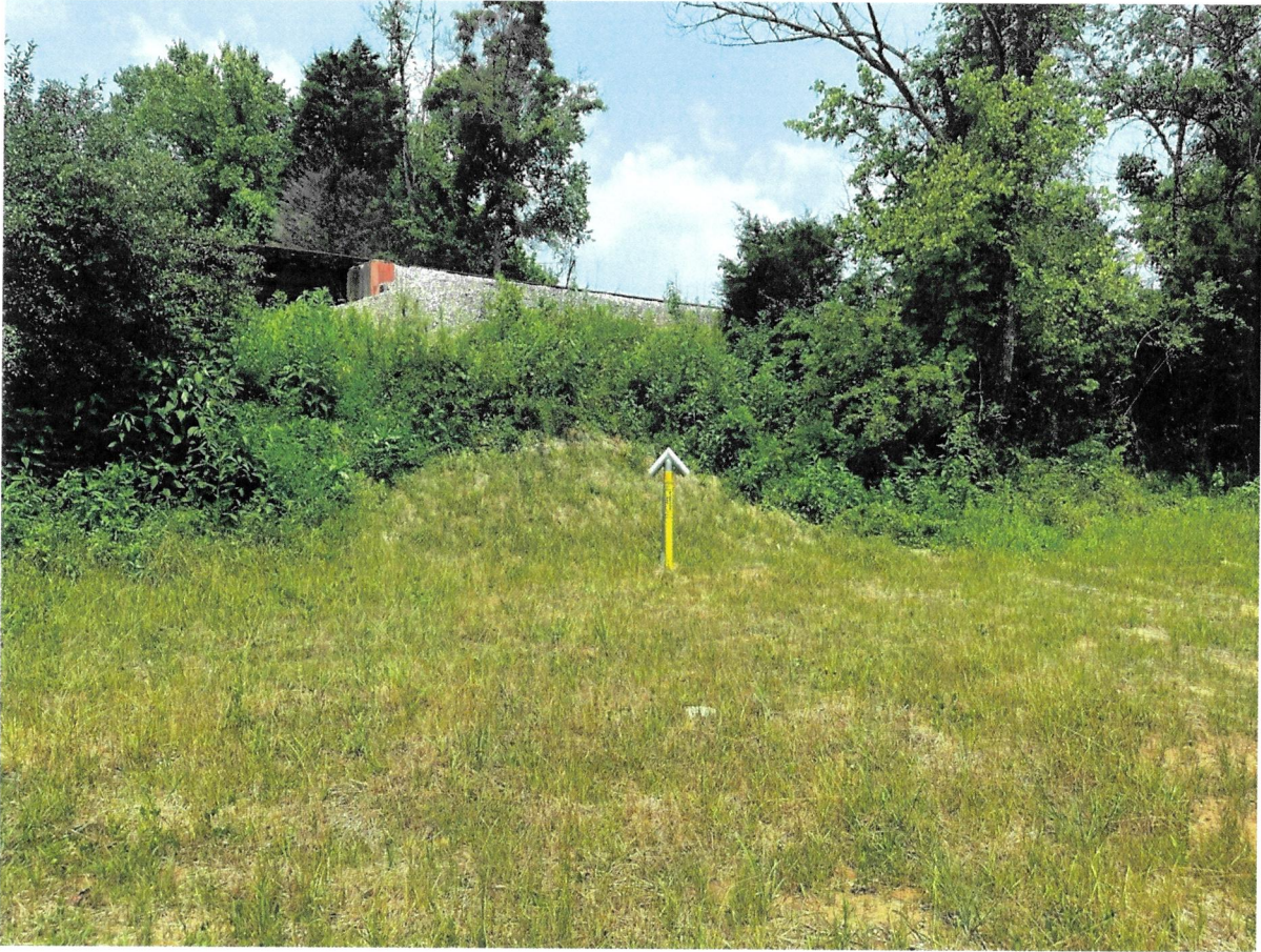
Figure 2. 70% Vegetation On North Side of Railroad - 7.26.23
