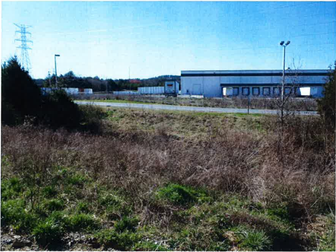
Unnamed Tributary looking west (GE Warehouse beyond)
