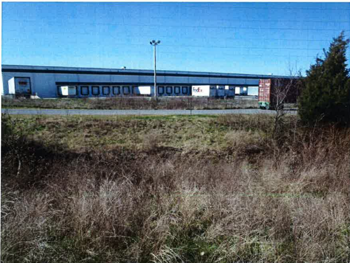
Unnamed Tributary looking west (GE Warehouse beyond)
