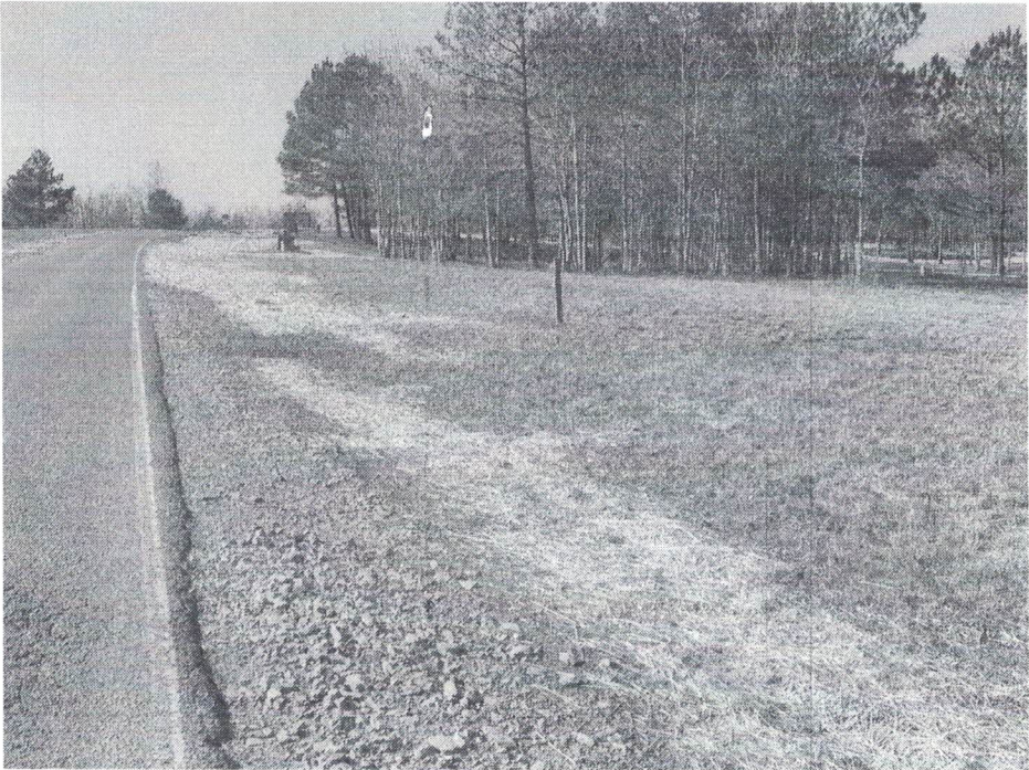
Photo 1: Outfall S59 Areas along the roadside have recently been stabilized with seed and straw. Photo Taken 2/26/2024
