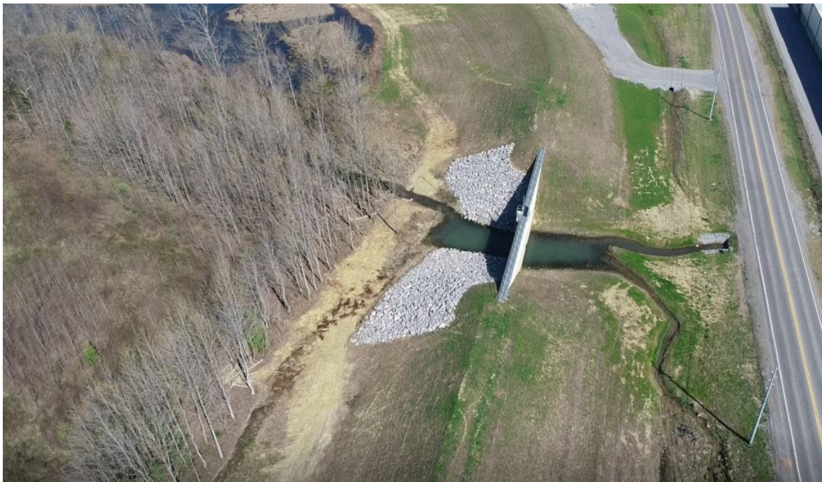
Large Flood wall STR-8 Relocation
