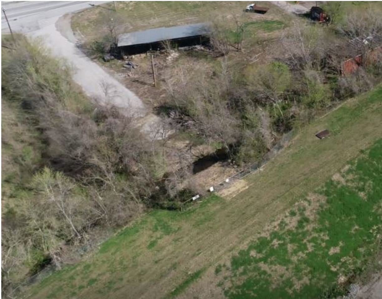
Bridge Removal Puzzle Fool Creek – A.O. Smith Entrance
