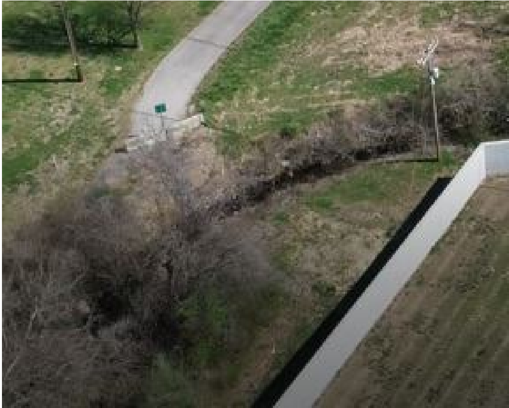
Bridge Removal Puzzle Fool Creek - Rhea Street
