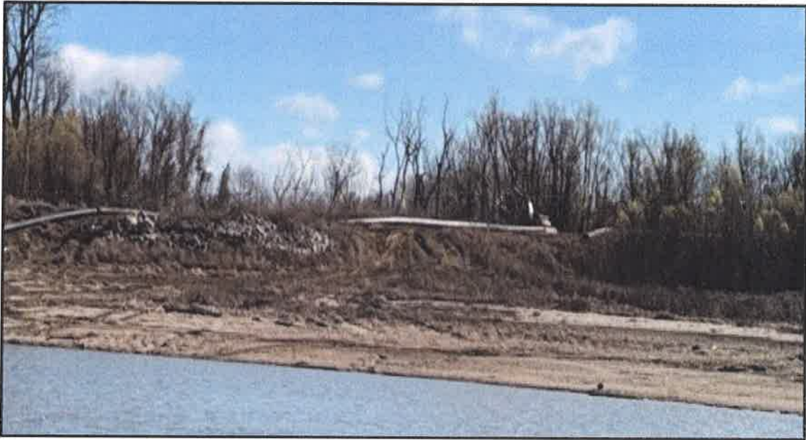
Piping system at Treasure Island.
