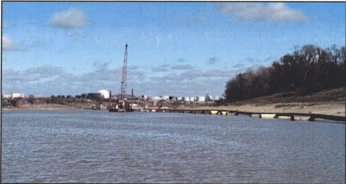
Piping system from dredging rig at the ADM Grain – Memphis facility transferring dredge material to Treasure Island.
