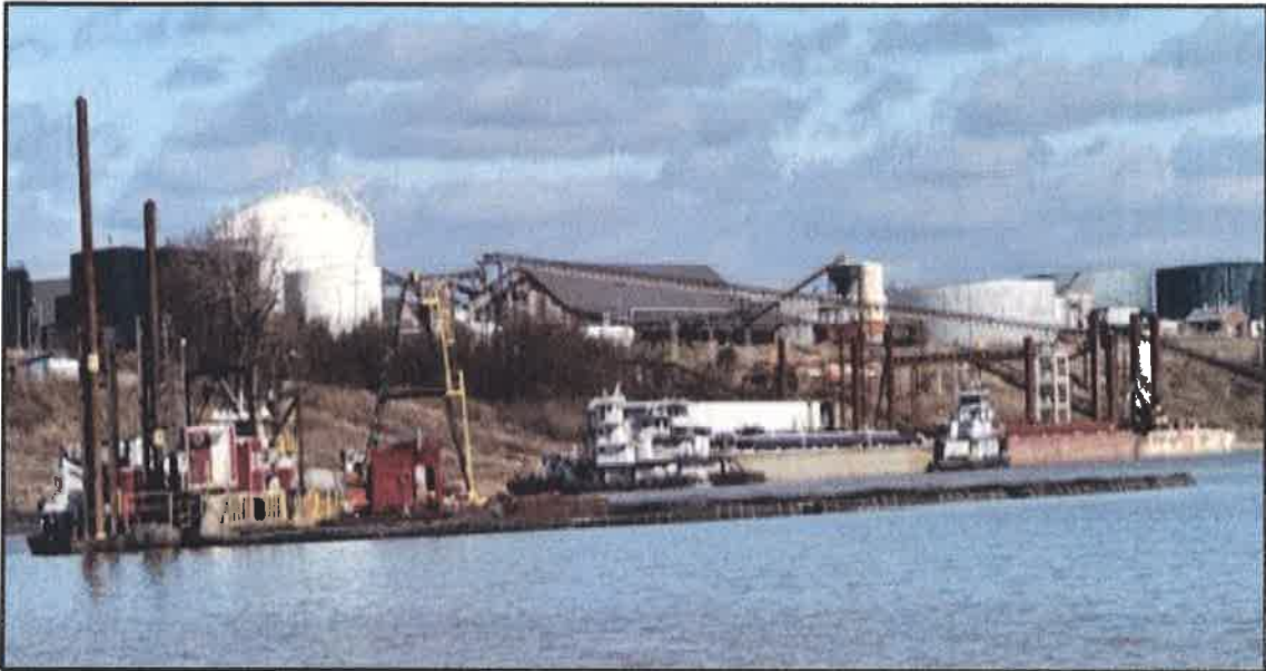
Piping system from dredging rig at the ADM Grain – Memphis facility transferring dredge material to Treasure Island.
